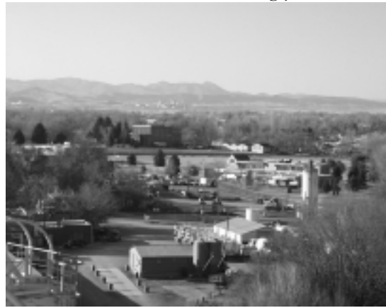
View Looking Northwest Towards the Old Power Plant
