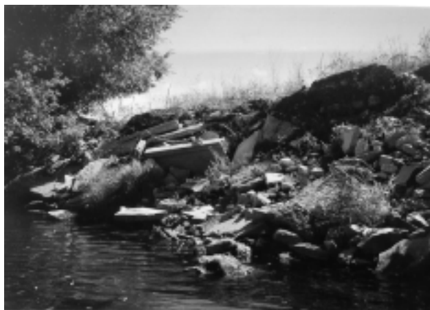
Typical Bank Condition in Corridor
