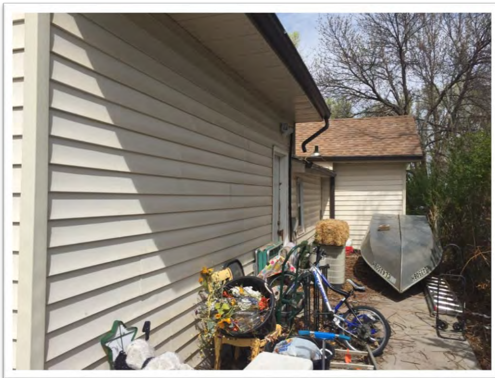
Building 1 North Elevation (upper) East Elevation (lower)
