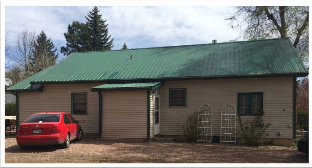
Building 1: Front (South) Elevation / Side (West) Elevation
