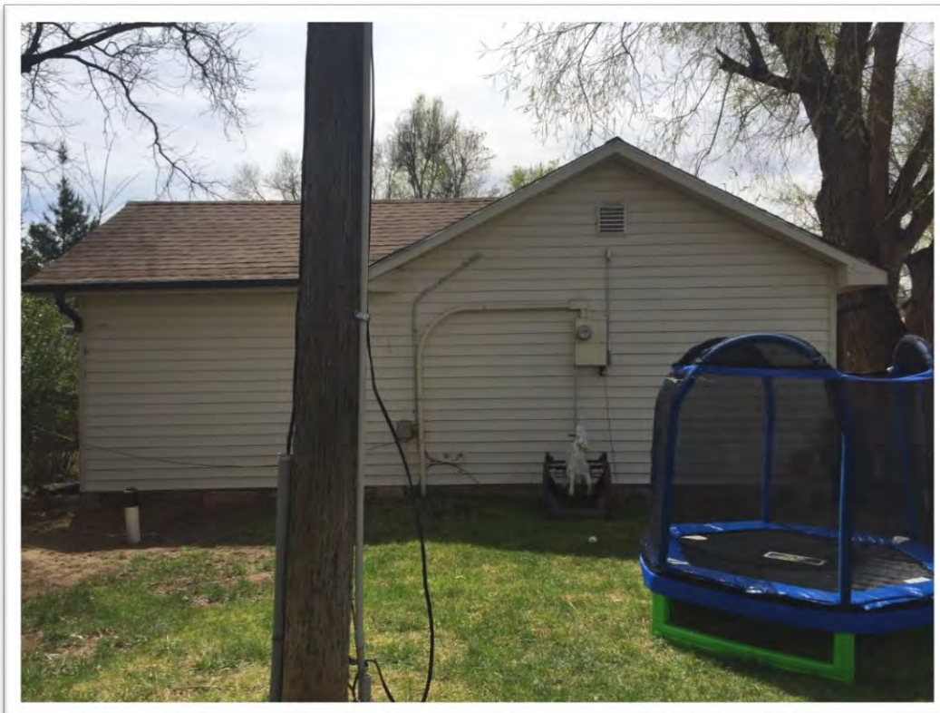
Building 3 Rear (North) Elevation
