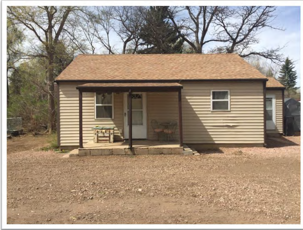
Building 2 Front (East) Elevation
