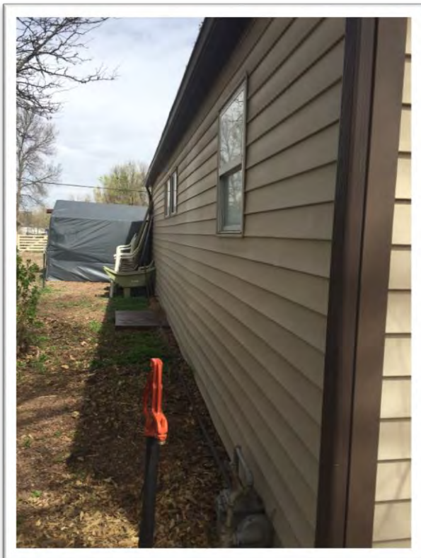
Building 2: Rear (West) Elevation
