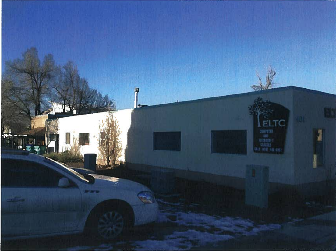
Southwest side of existing ELTC (401 Linden) building.
