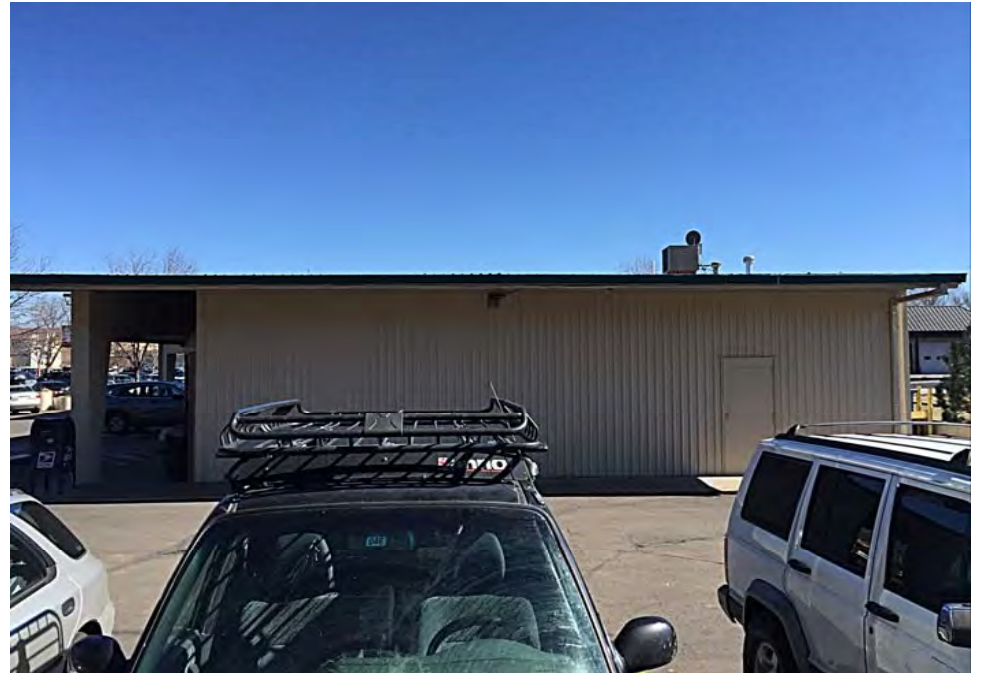
East Building - West Elevation
