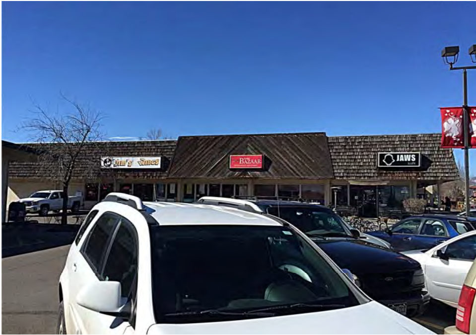
West Building - East Elevation
