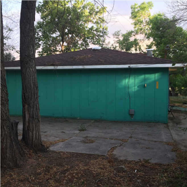
North elevation of residence (facing Drake)
