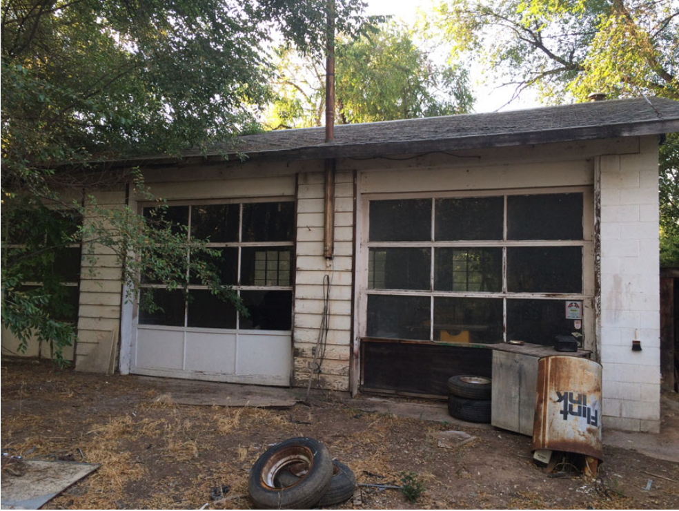
South elevation of Garage/Shop
