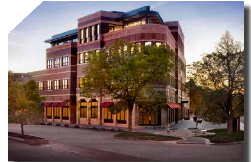
The taller corner marks the important gateway at the Walnut and Chestnut St. intersection and balances the building scale against the Mitchell Building .
