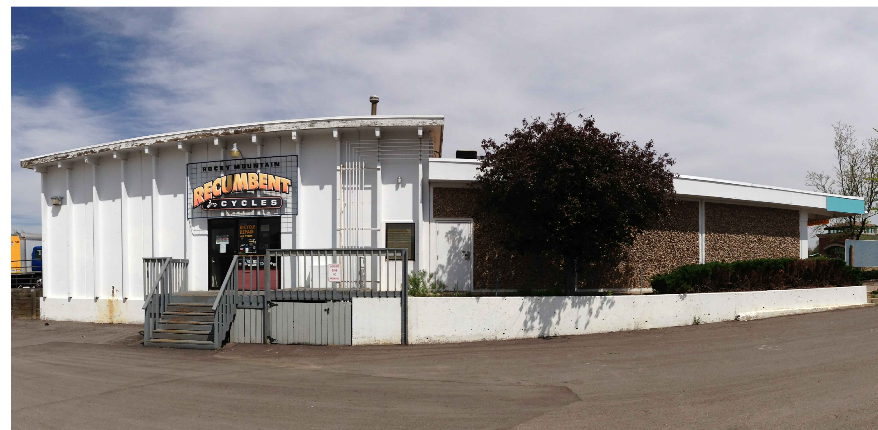
WEST SIDE VIEW
