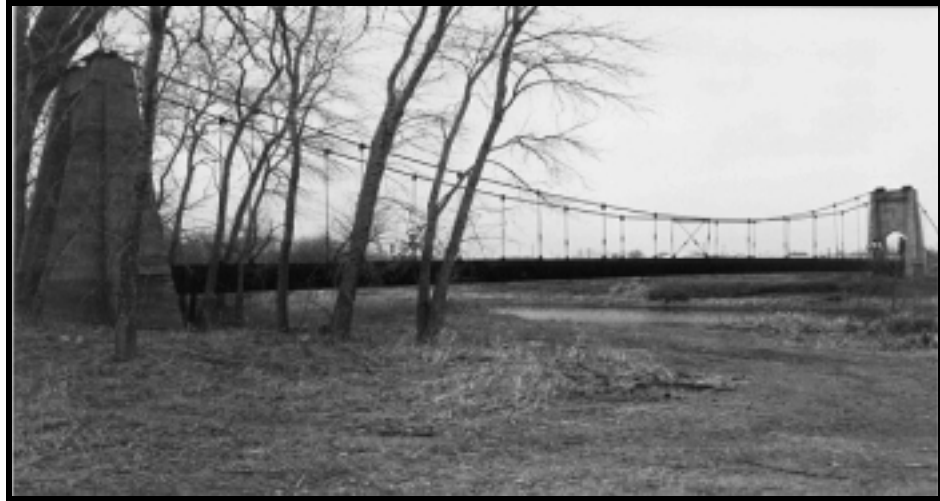
Great Western Sugar Effluent Flume
