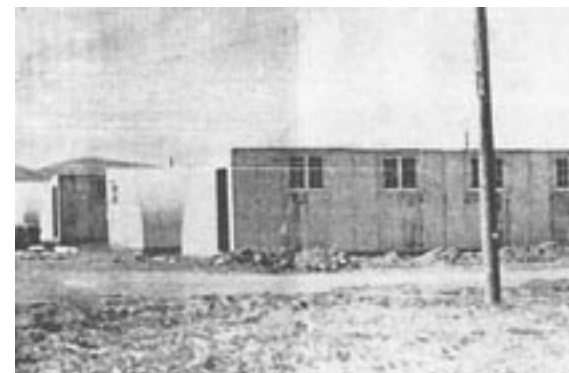
Figure 11. This photograph, which appeared in the Rocky Mountain Collegian as Veterans' Village was assembled, shows the placement of the Montgomery Ward half Quonset huts. ( Rocky Mountain Collegian , 28 February 1946, p. 1)
