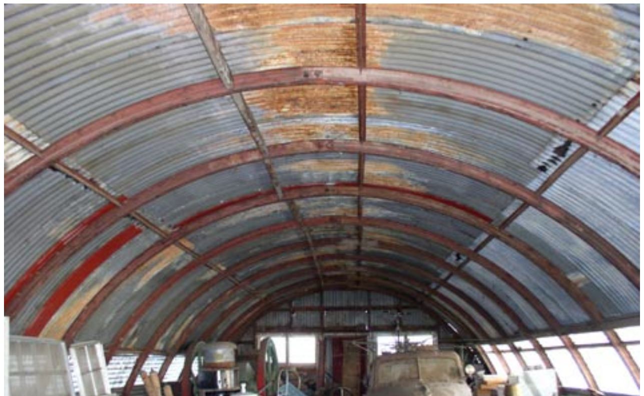
Figure 6. The interior view of a 20-by-48-foot, war-surplus Quonset reveals the original arch-rib design Dejongh developed at Quonset Point, except that the original perflins are steel rather than wood. Colorado A&M (CSU) first acquired this particular Quonset for veteran-student housing. It is now located at the Swetsville Zoo, 4801 East Harmony Road. (Photo by the author)
