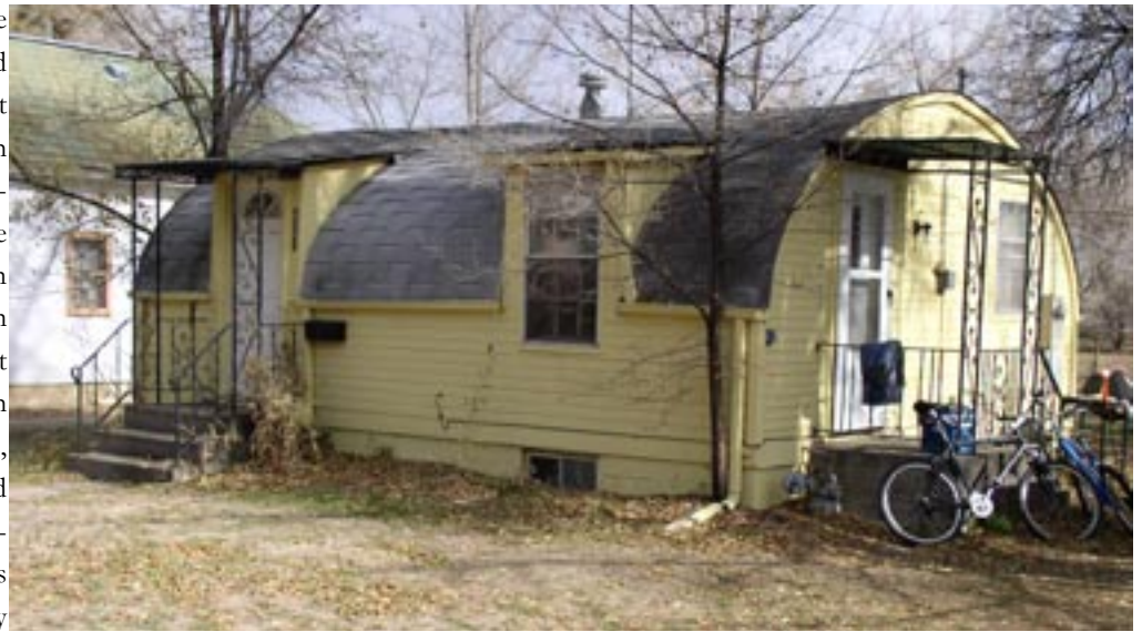
Figure 15 and 16. Fort Collins hosts two wood-frame, kit-built Quonset hut cottages. Both were built in 1947. This one, located on Lesser Drive, retains many of its original details. The Fort Collins Gambles store began advertising these structures (below) in the summer of 1946. (Photo by the author; Fort Collins Coloradoan , 7 July 1946, p. 7)
