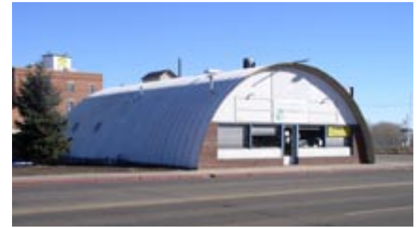
Figure 17. This Quonset hut, at 416 Jefferson Street, differs from the other huts on the same street because its structural support system and exterior cladding are the same component. (Photo by the author)
