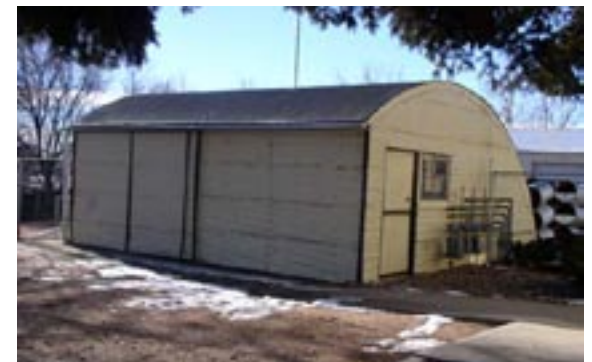
Figure 18. Two-thirds Quonset huts, in this case a Stran-Steel Quonset 24, provide a flat side for the installation of doors larger than could be accommodated in the ends. This structure is located at 413 U.S. Highway 287 North. (Photo by the author)
