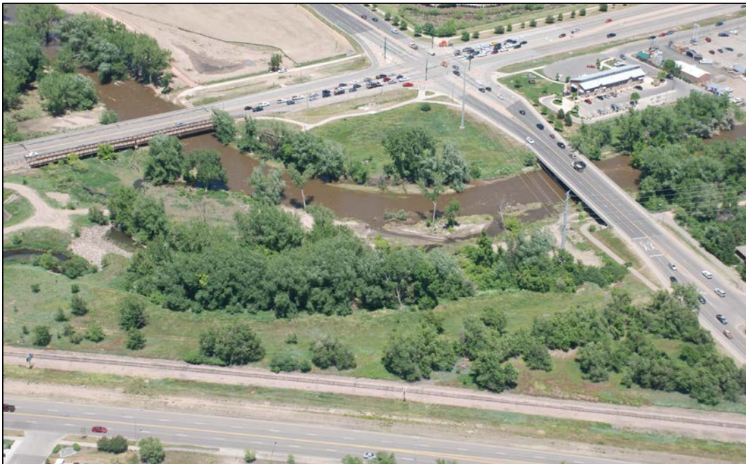
Figure IV.3 Bank stabilization, confinement at bridge underpasses, and development encroachment into the floodplain is observed where the Poudre travels under Mulberry St. and Lemay Ave. bridges and parallel to Riverside Ave.
