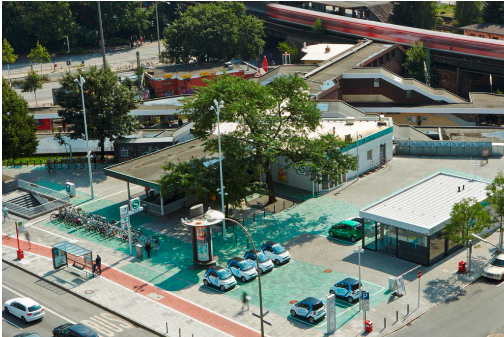
Figure 20 – Mobility hub in Hamburg, Germany (see Figure 21 for description)
