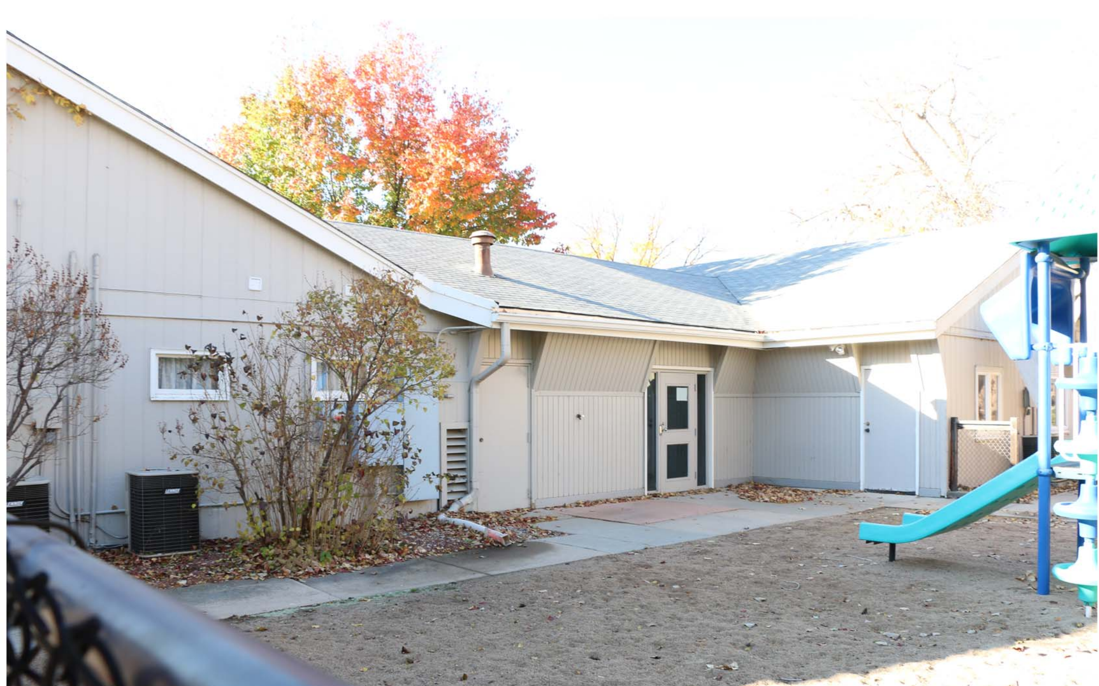
MAIN BUILDING- NORTH SIDE (BACK)
