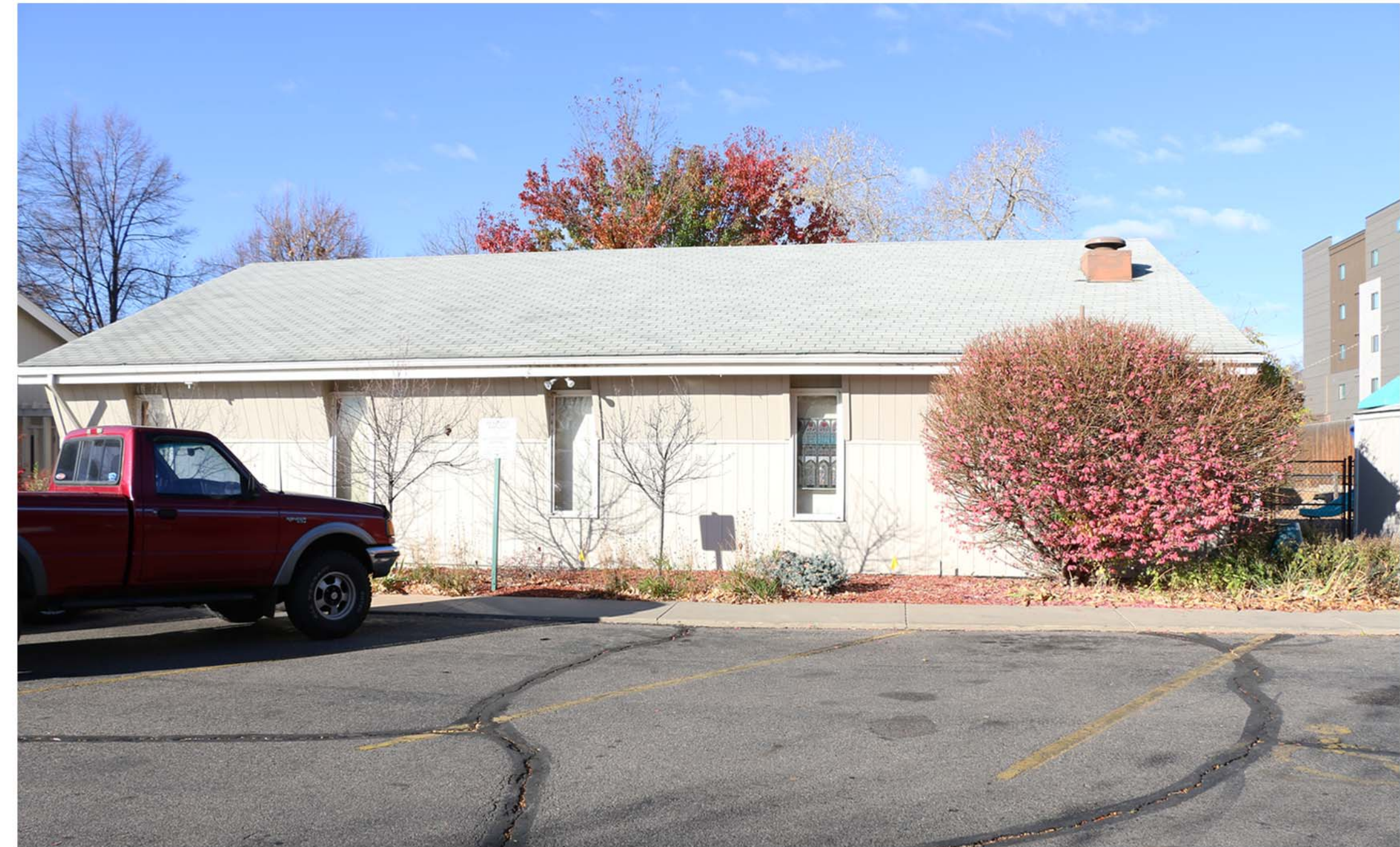
MAIN BUILDING- EAST SIDE
