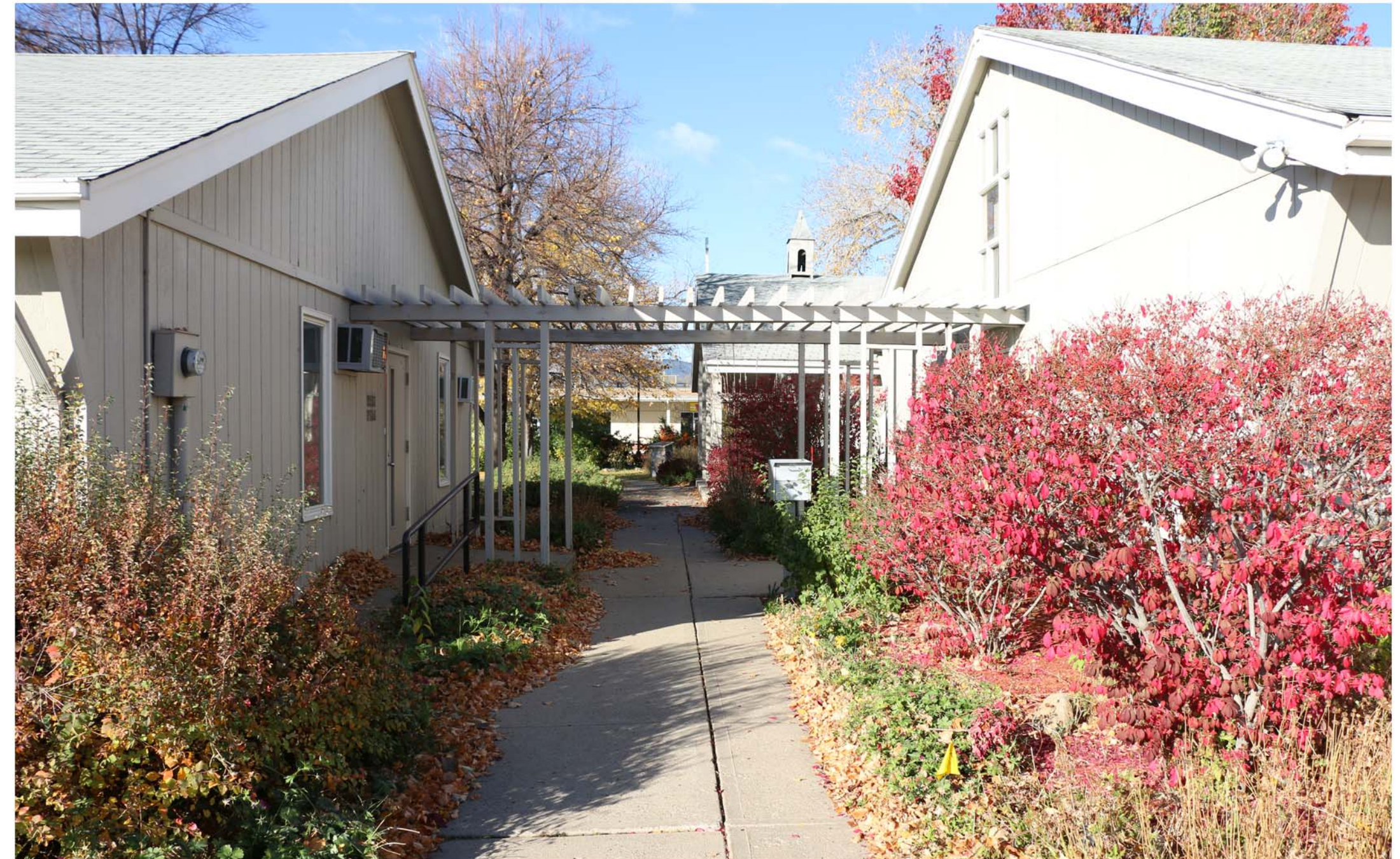
SOUTH SIDE OF MAIN BUILDING & NORTH SIDE OF ACCESSORY BUILDING
