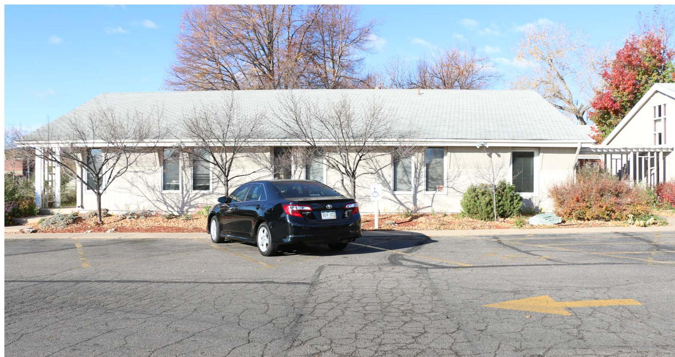
ACCESSORY BUILDING- EAST SIDE
