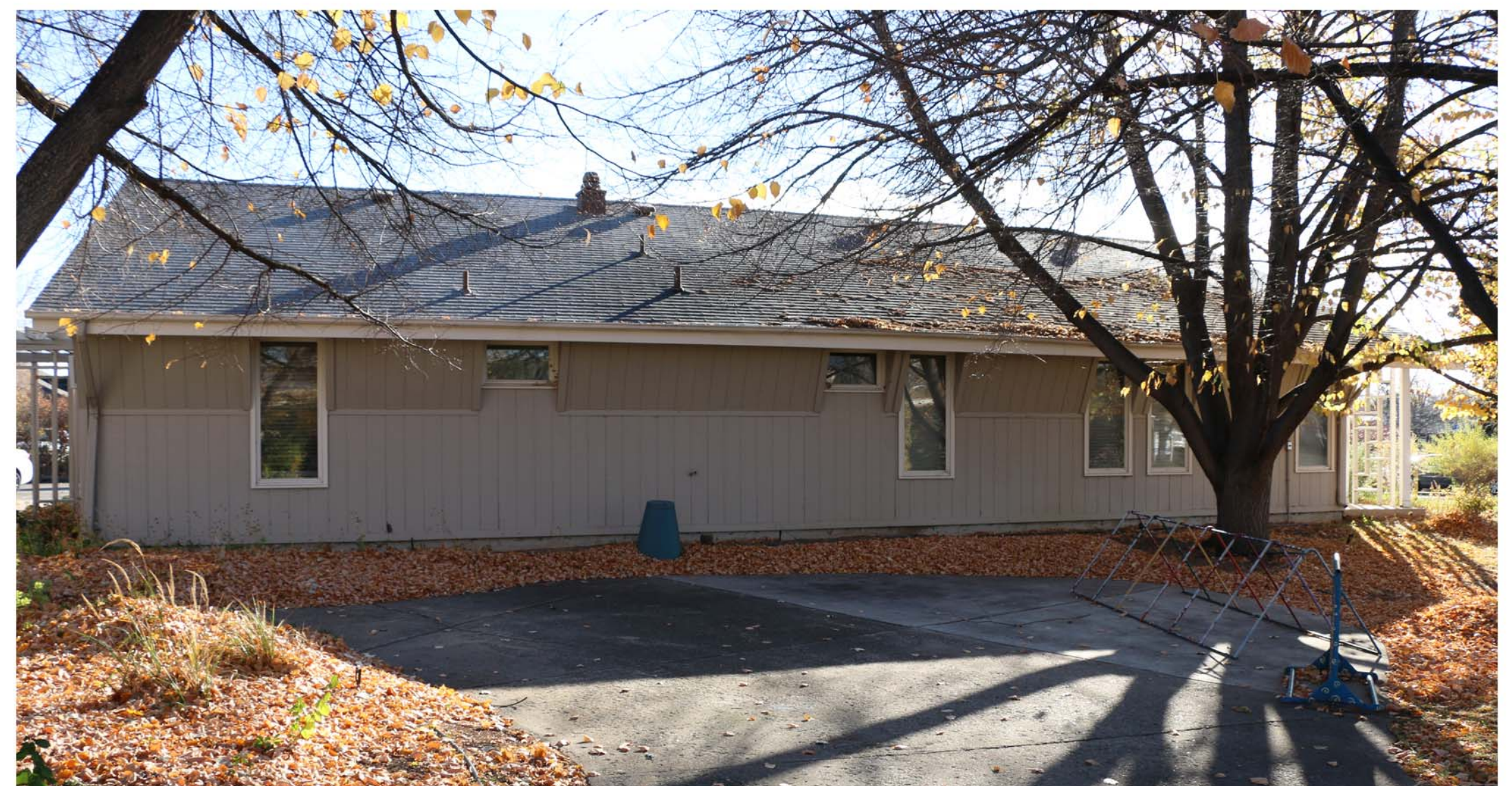
ACCESSORY BUILDING- WEST SIDE
