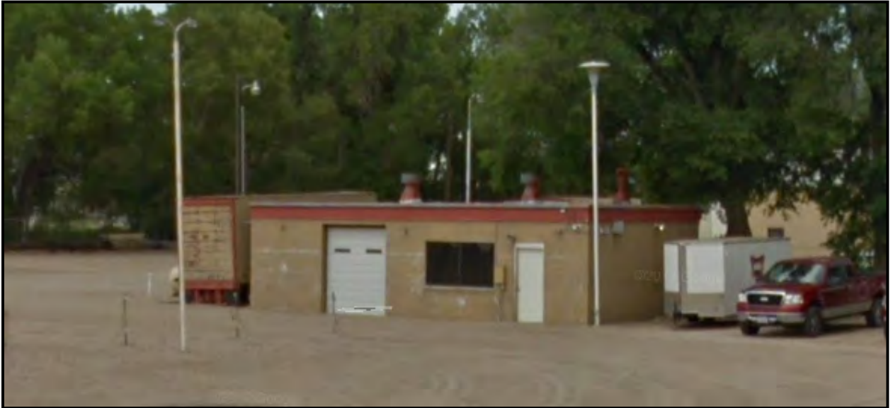
2. Garage #2 – Masonry block, 800 SF, built 1967
