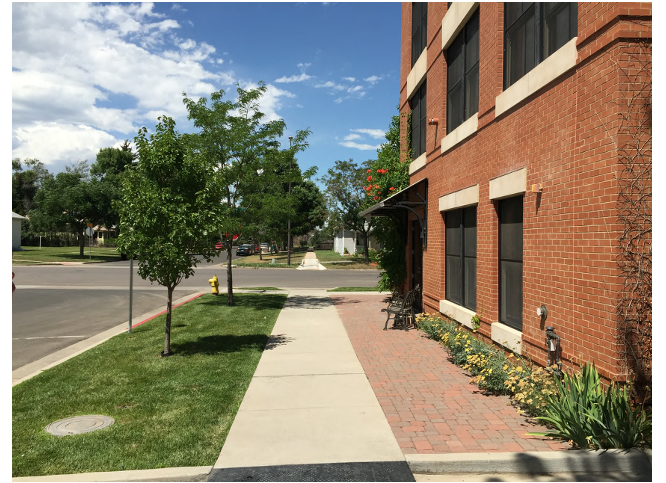
CHERRY STREET LOFTS STREETScape AT THE INTERSECTION OF CHERRY AND MELDRUM
