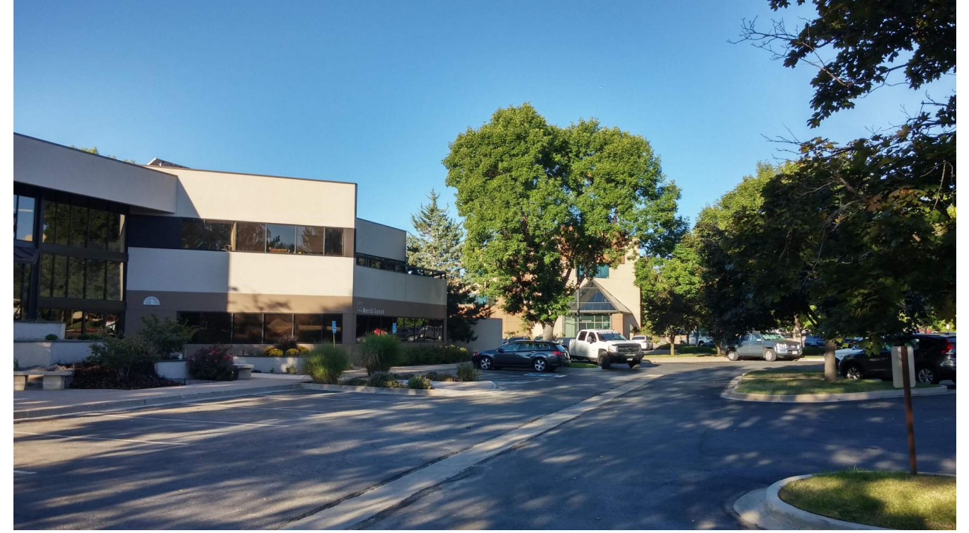
EXISTING BUILDING - NORTHEAST VIEW FROM LOT / STANFORD RD
