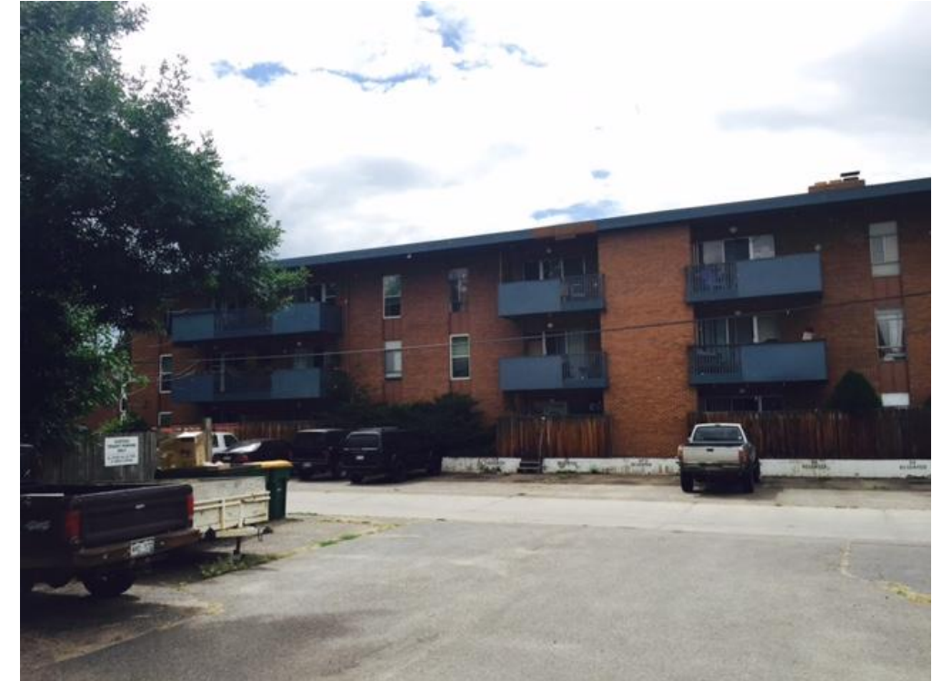
3-story apartment complex across alley immediately west
