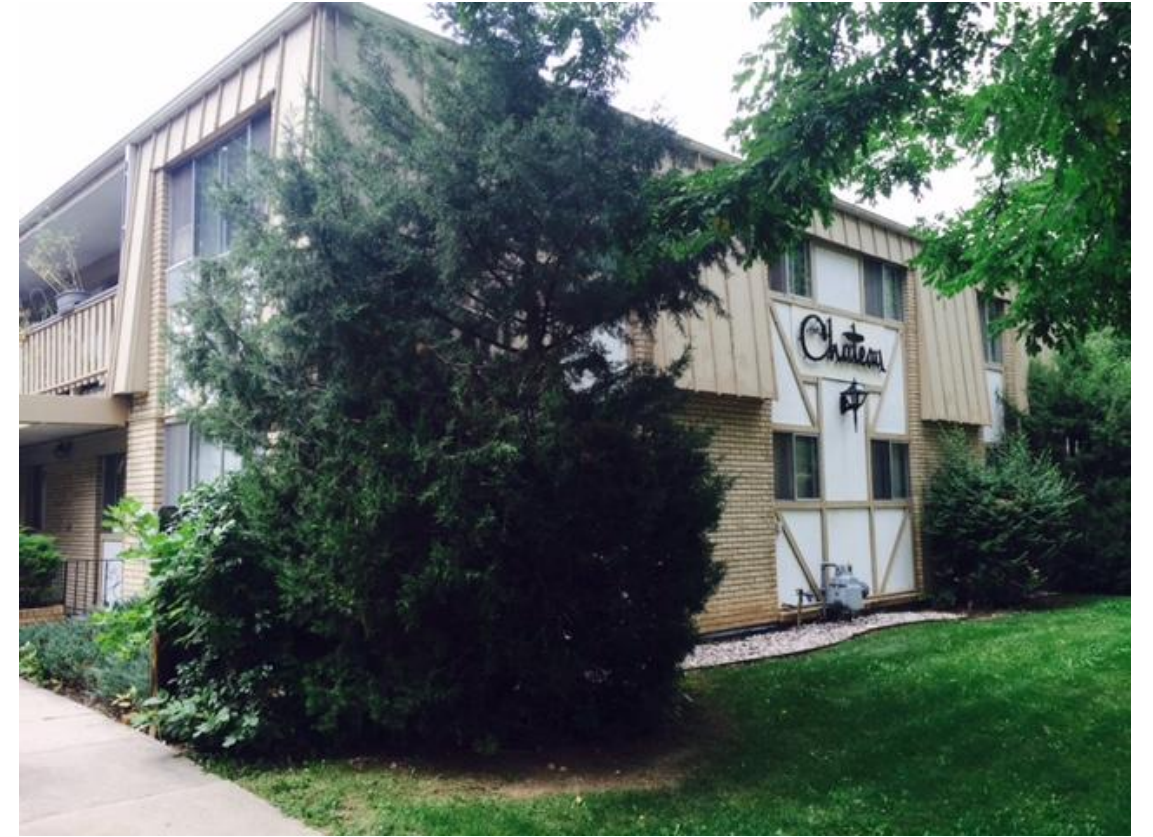
2-story Chateau Apartment complex immediately north
