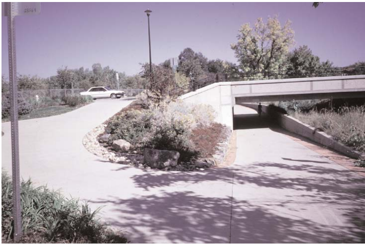
Cross Street Accessibility
