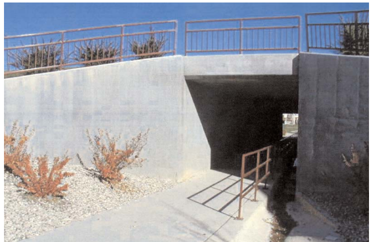
Protective Railing Between Usable Path and Drainage Facility
