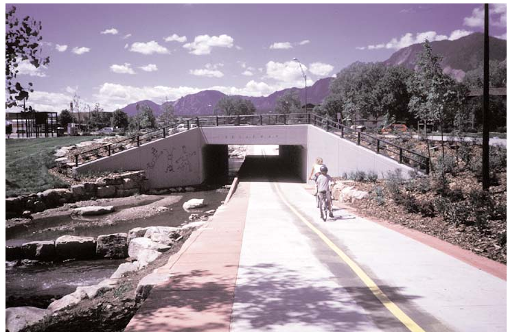
Structure with Drainage Facility
