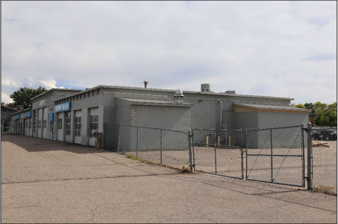
Figure 13: Feature 1, north and west elevations, view southeast (Image #7231, R. Shields, 10/3/2023).
