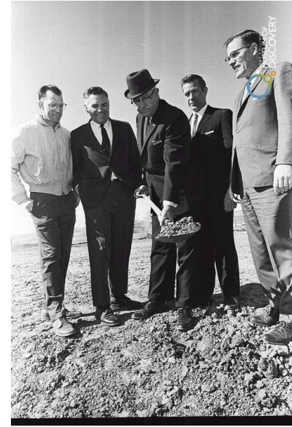
Ghent Motors Ground-breaking, March 9, 1966
