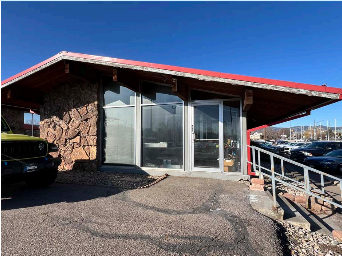
43. East Elevation - Entrance and office area of the small garage. Image courtesy of BEE. 2024.
