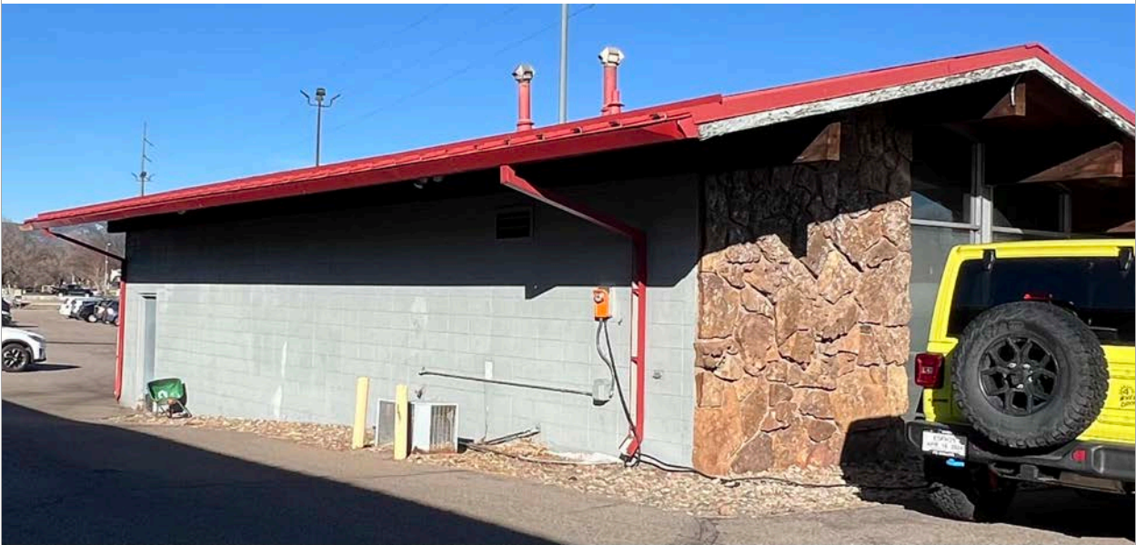
47. South Elevation - Small door at the service area. Image courtesy of BEE. 2024.
