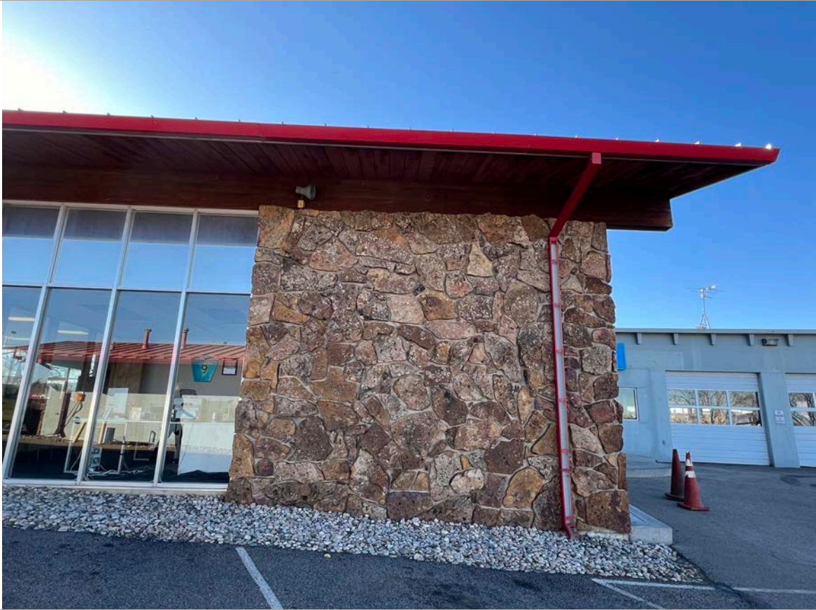
13. North Elevation - to NW Corner of showroom. Image courtesy of BEE. 2024.
