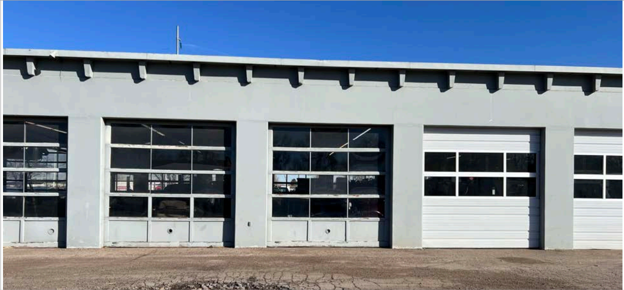
34. South Elevation - Service center, bays 3-7. Image courtesy of BEE. 2024.
