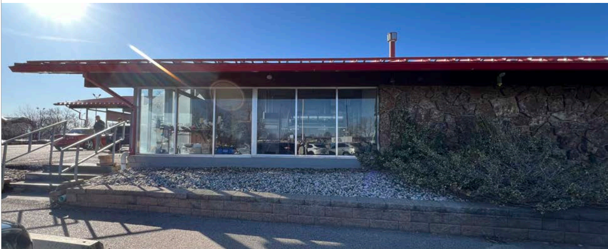
44. North Elevation - Entrance and office area of the small garage on photo left, service area at photo right. Image courtesy of BEE. 2024.
