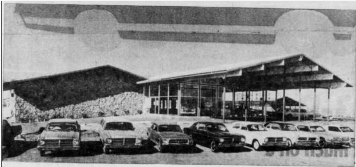
Figure 2: 2601 S. College facade. Image clipped from Coloradoan . October 26, 1966.
