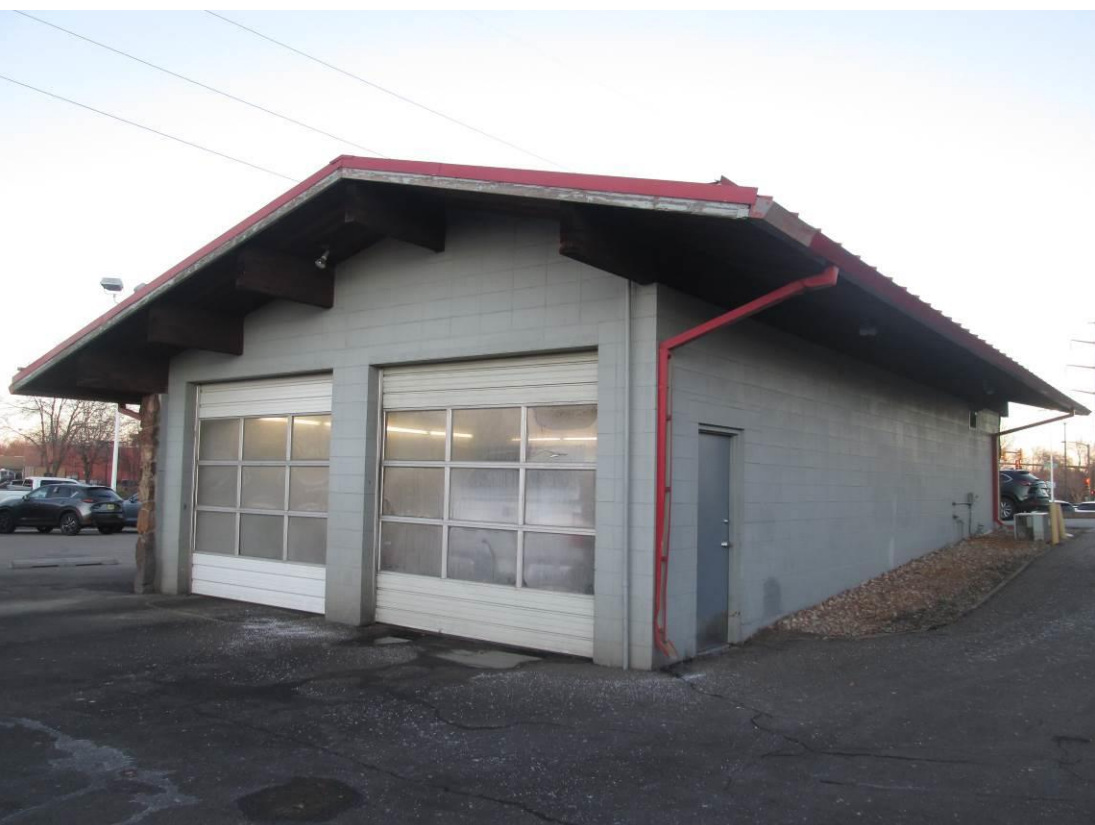
5LR.14283 – Spradley-Barr – Used Car Sales. (Bldg. B) Western and southern elevations. Looking southwest. December 2017. Image 5LR.14283i.
