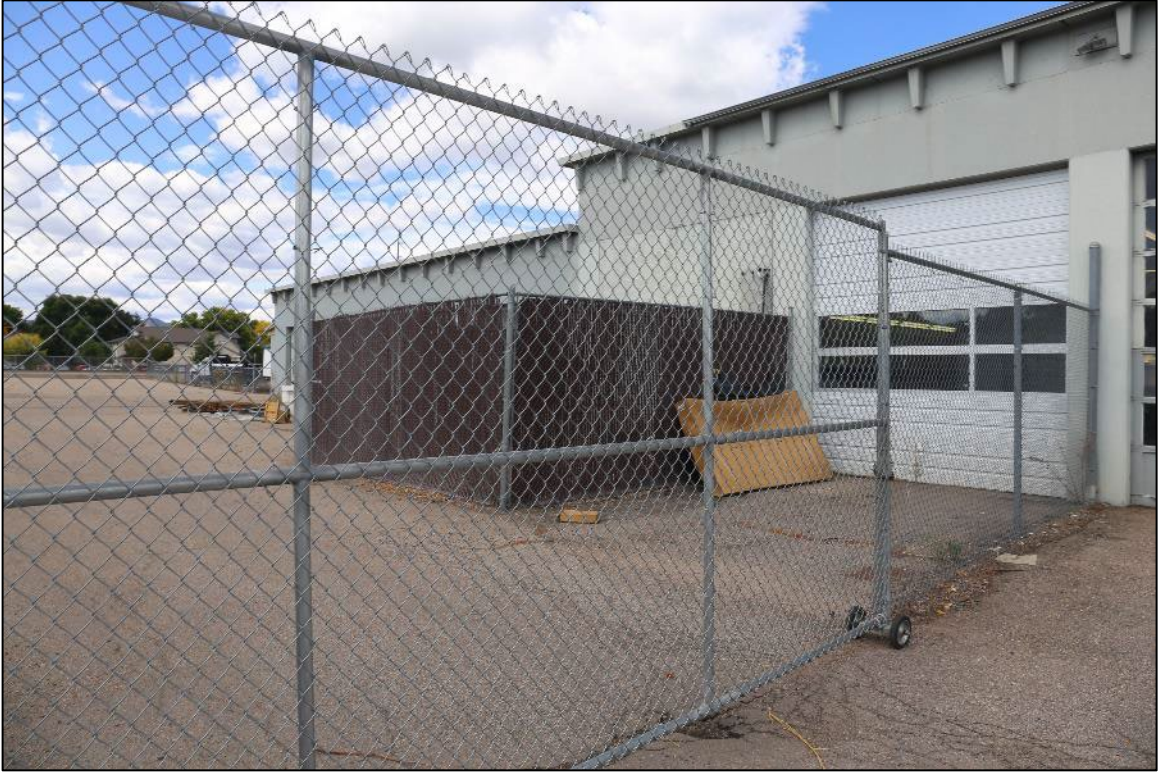
Figure 14: Feature 1, west end of south elevation, view northwest (Image #7246, R. Schields, 10/3/2023).
