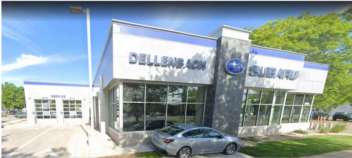
74. Subaru dealership, 3103 South College Ave. Built in 1973, not eligible for landmarking per the City of Fort Collins Historic Resources Planning Map. Image courtesy of BEE. 2024.
