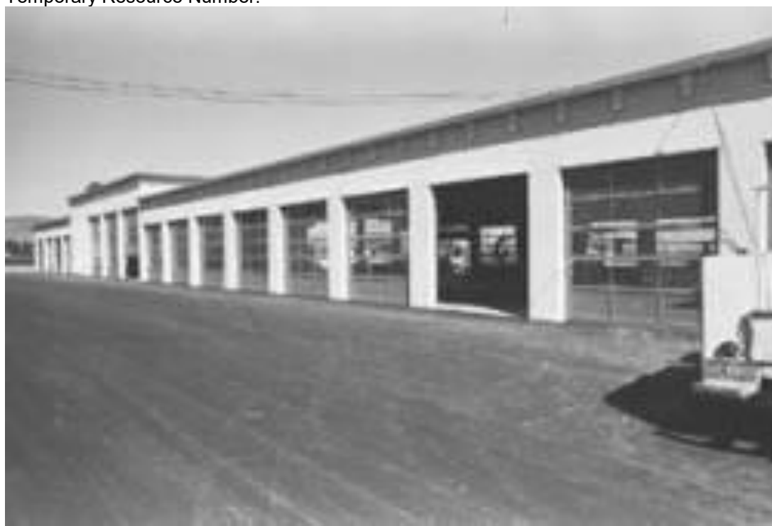
Ghents Motors. Photos showing the southern elevation of the Service Bay Section with original rolling garage doors. Photos taken September 1, 1966 From Coloradoan Collection, Fort Collins Museum of Discovery.
