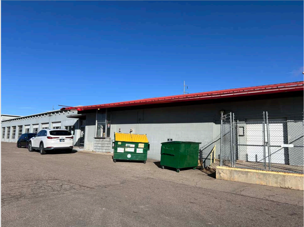
39. South Elevation - Showroom, dumpsters, door at stairs, and loading dock with roll-up door. Image courtesy of BEE. 2024.
