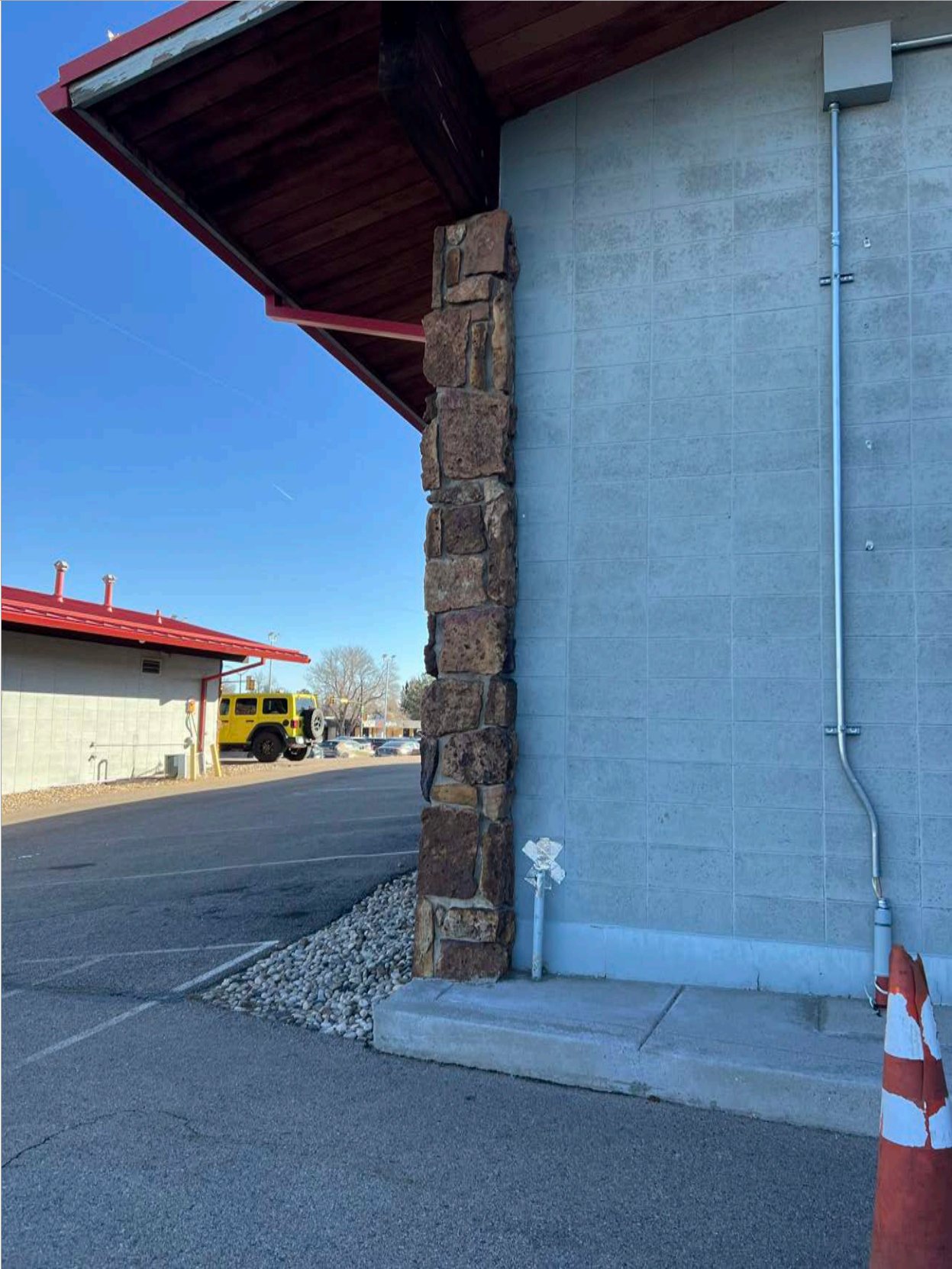
24. West Elevation - NW corner of the Showroom. Image courtesy of BEE. 2024.
