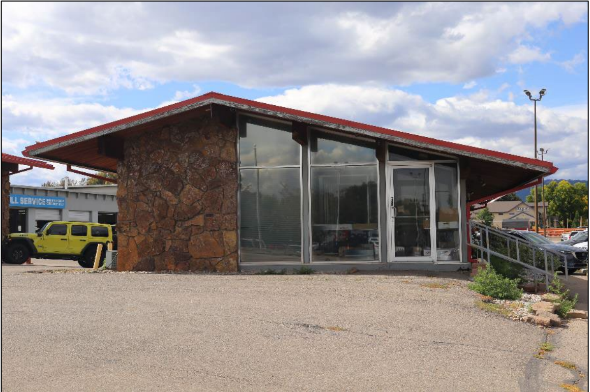
Figure 20: Feature 2, east-northeast elevation, view west (Image #7205, R. Schields, 10/3/2023).
