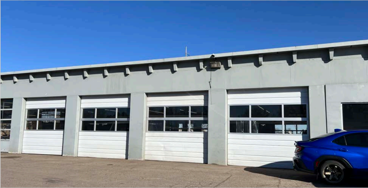
35. South Elevation - Service center, bays 1-5. Image courtesy of BEE. 2024.
