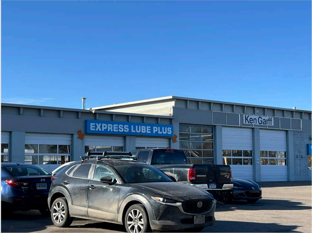
17. North Elevation - Service center, bays 5-8. Image courtesy of BEE. 2024.
