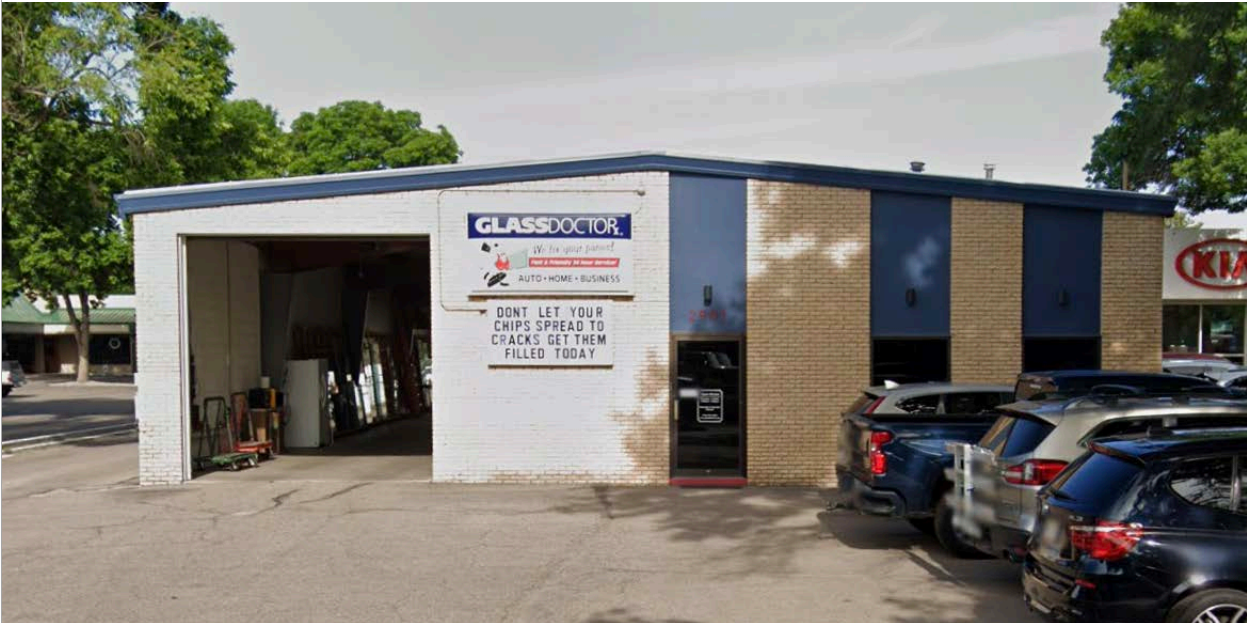
71. Glass Doctor, 2901 South College Ave, date of construction unknown, not eligible for landmarking per the City of Fort Collins Historic Resources Planning Map. Image courtesy of BEE. 2024.
