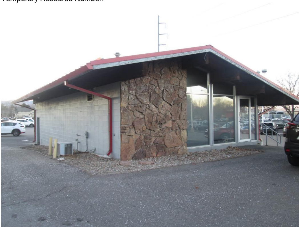
5LR.14283 – Spradley-Barr – Used Car Sales (Bldg. B) Eastern and southern elevations. Looking northeast. December 2017. Image 5LR.14283j.
