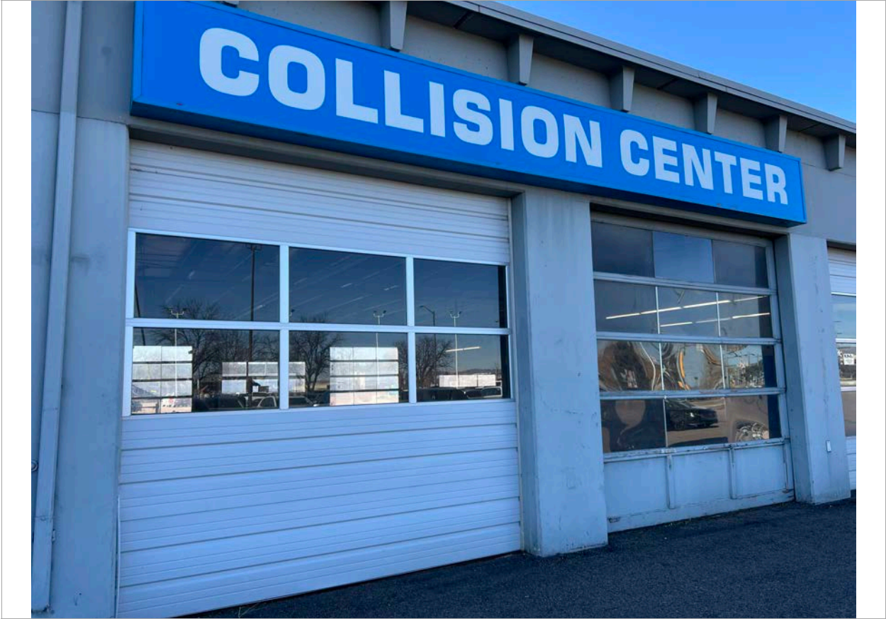
20. North Elevation - Service center, bays 12 and 13. Note the door on bay 13 is original. Image courtesy of BEE. 2024.
