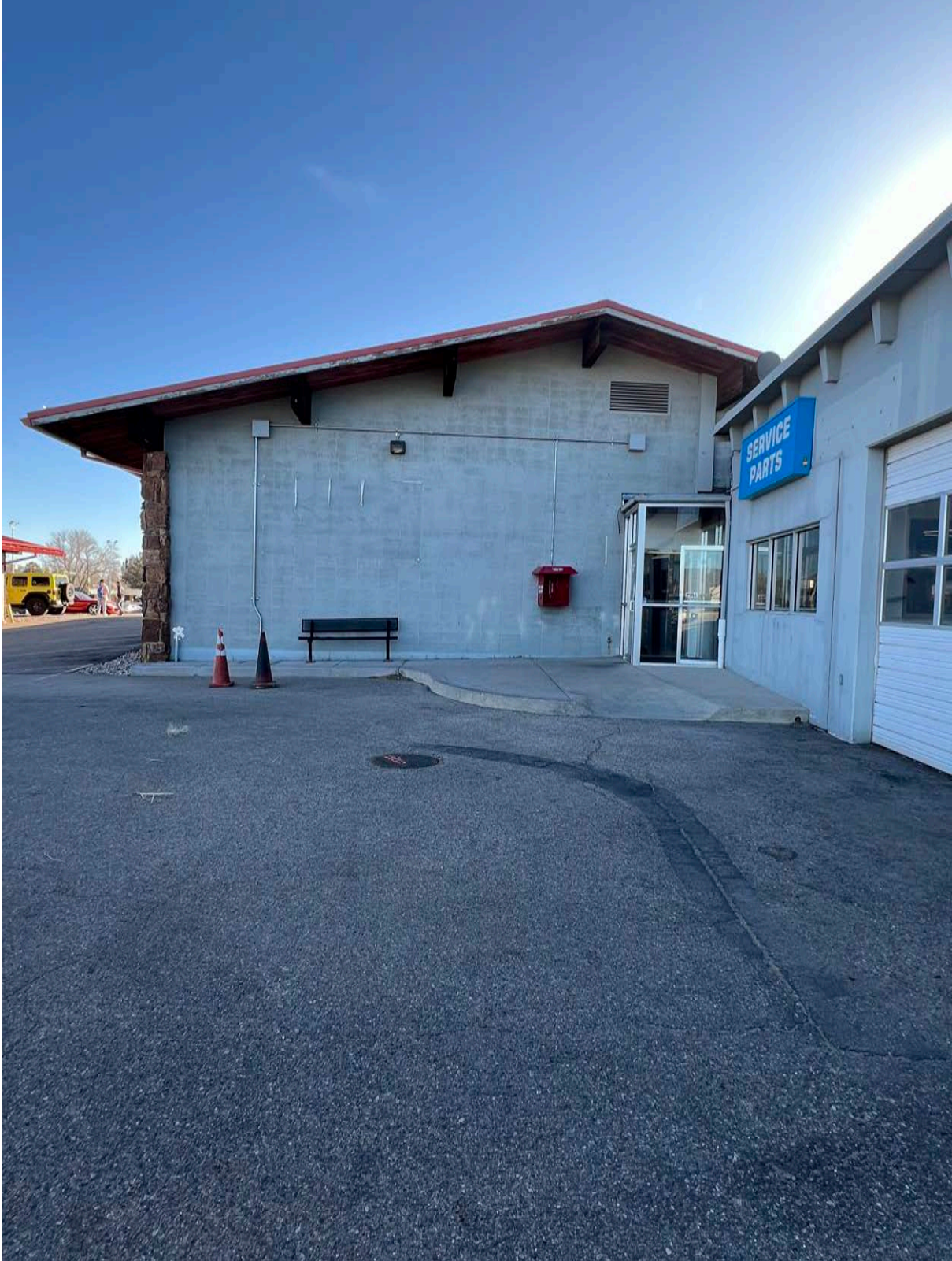
23. West Elevation - Back wall of the Showroom. Image courtesy of BEE. 2024.
