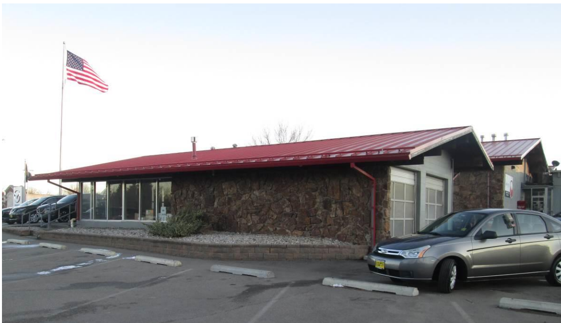
5LR.14283 – Spradley-Barr – Used Car Sales (Bldg. B) Northern elevation. Looking southeast. December 2017. Image 5LR.14283k.
