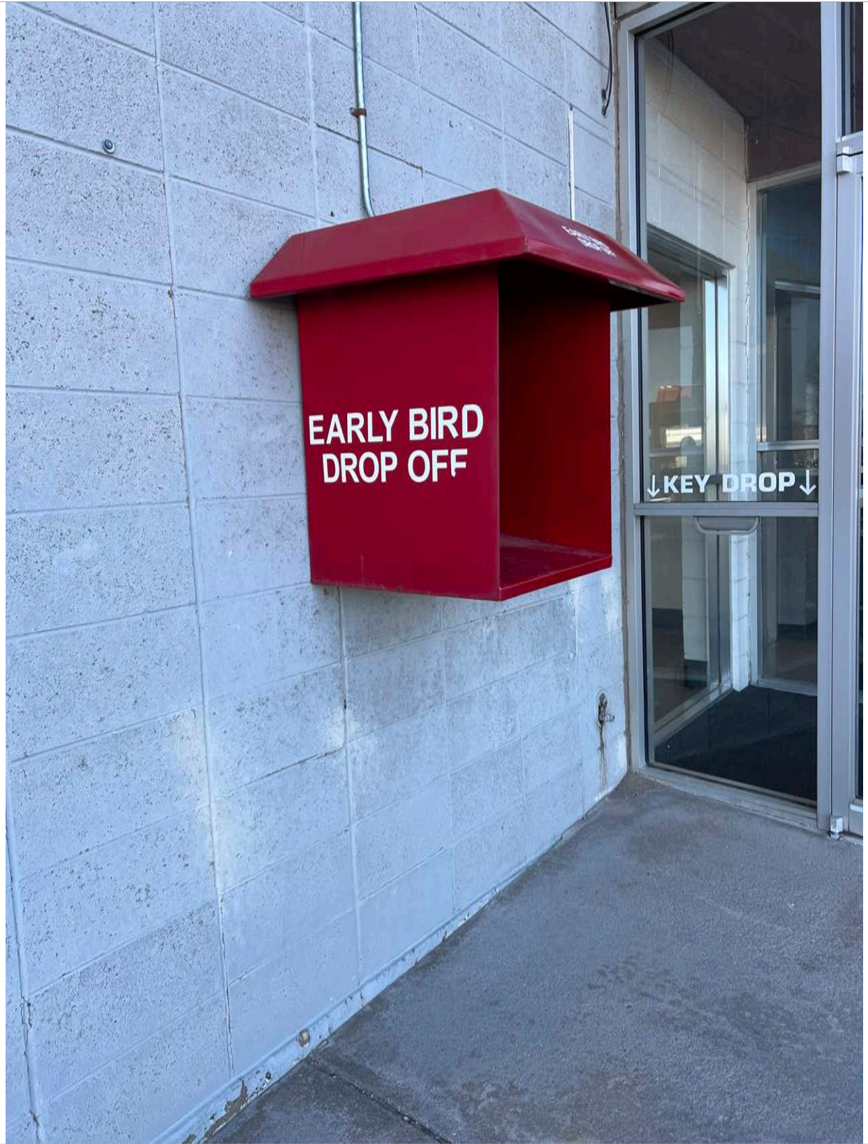
31. West elevation - Detail of key drop. Image courtesy of BEE. 2024.
