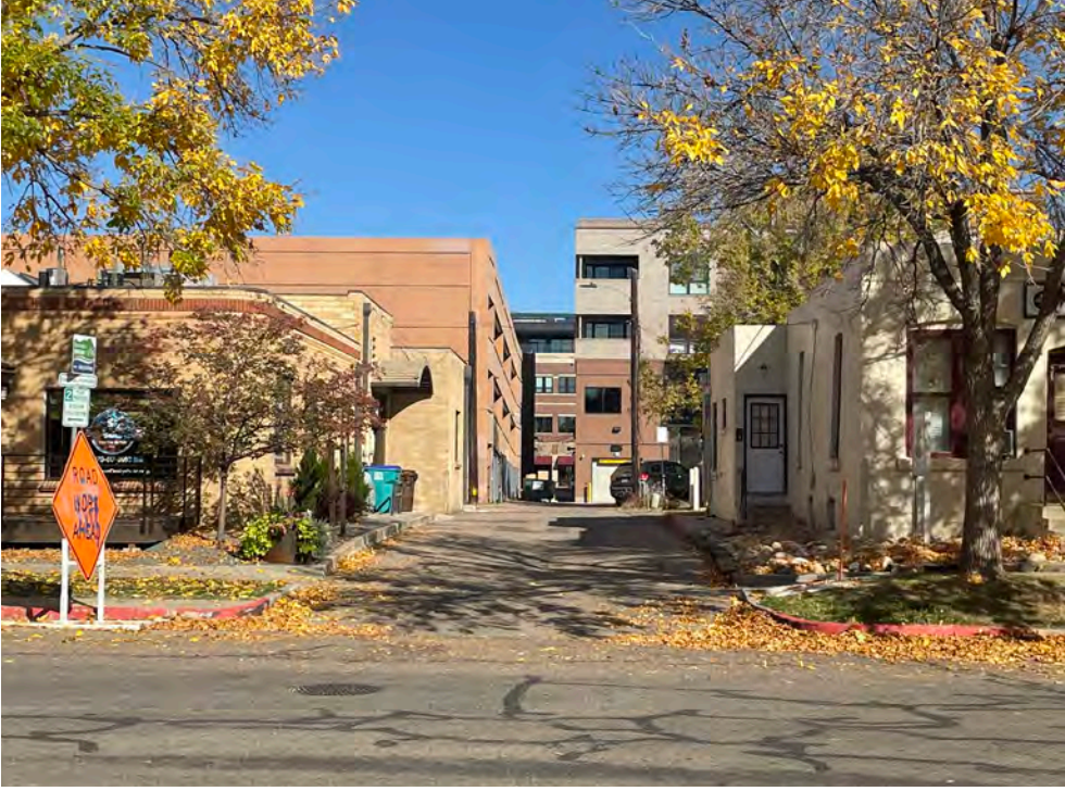
LOOKING NORTH AT ALLEY PROPERTY LINE
