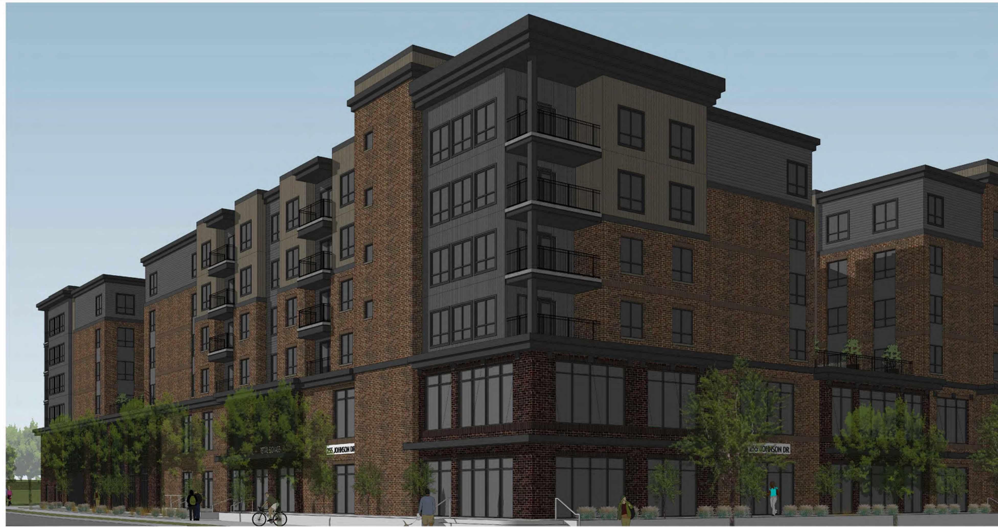
MAIN ENTRANCE, LOOKING SOUTH
