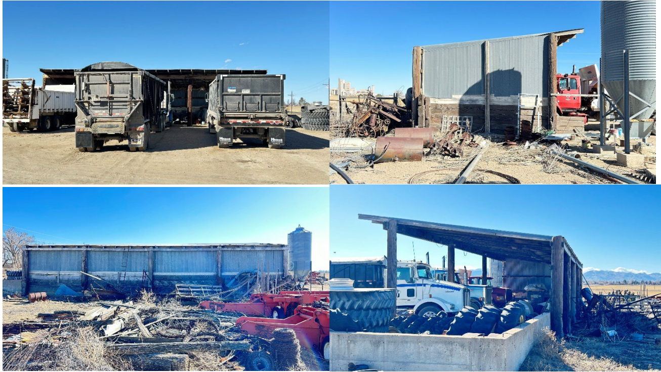
Building ID 505 Farm utility loading shed, pole building, built in 1970, low quality, 1.044 sf Age: 54 years
