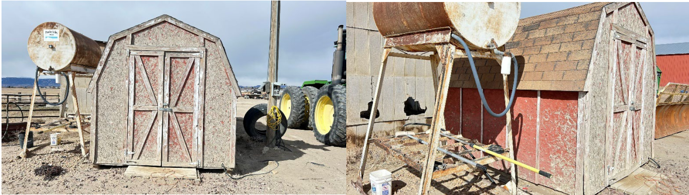
Building ID 507 Tool shed, wood frame, built in 1970, low quality, 168 sf Age: 54 years
