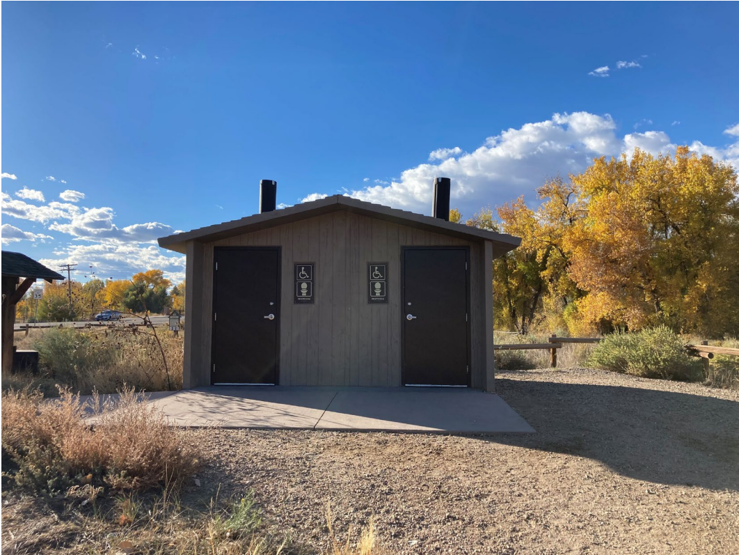
Double vault toilet
