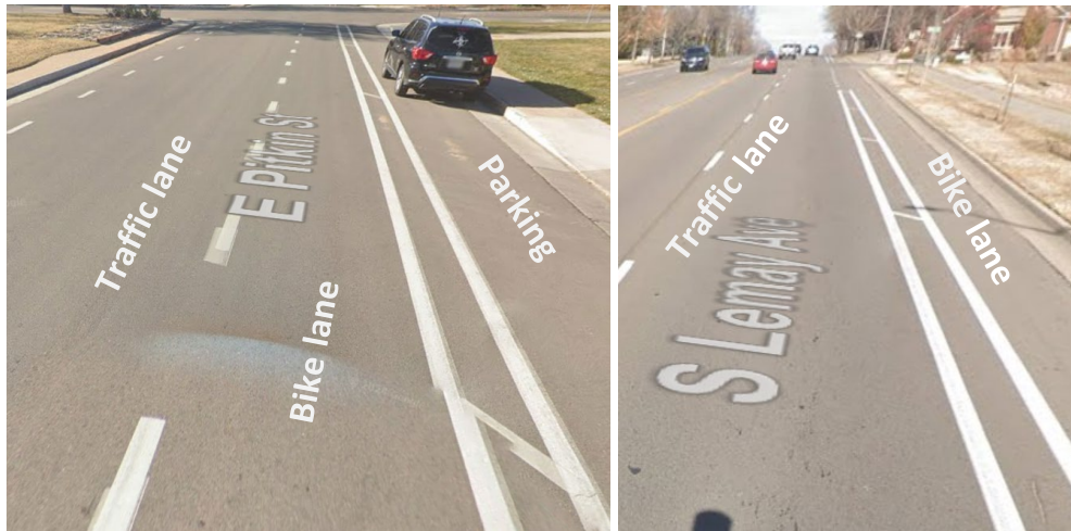
Figure 3. Striping on advisory lanes (left) versus on a buffered bike lane (right).
