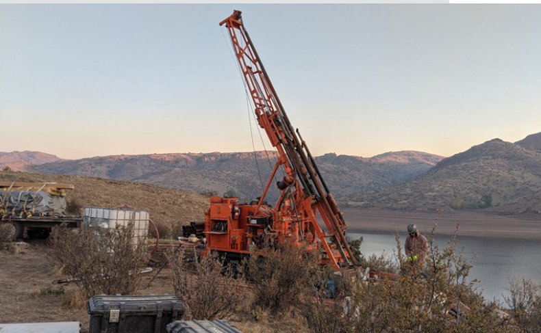
Drilling to evaluate ground conditions for the enlarged dam
