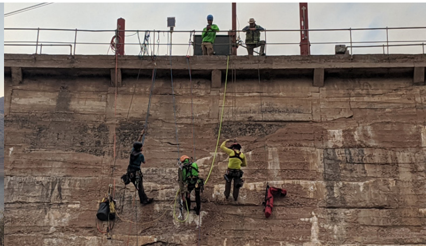
Extracting cores to evaluate structural integrity of the 111-year-old dam
