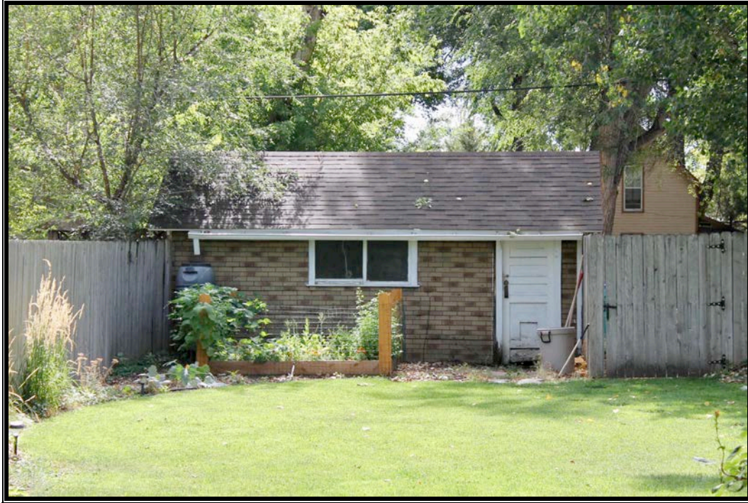
View of the Garage from the Rear Yard, View to the South
