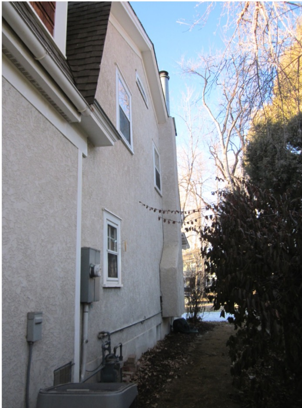
Reidhead: East elevation
