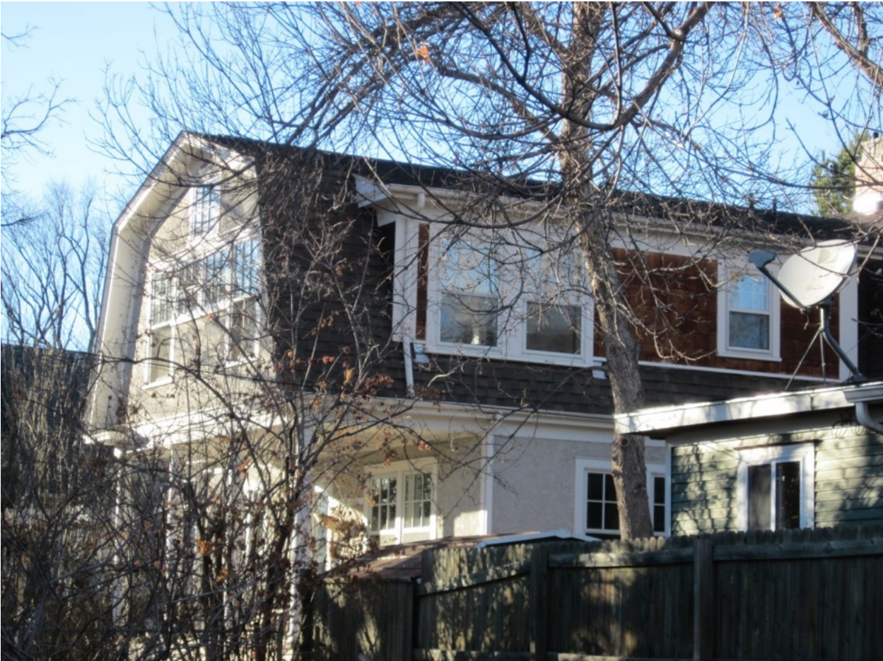
Reidhead: South and east elevation, addition
