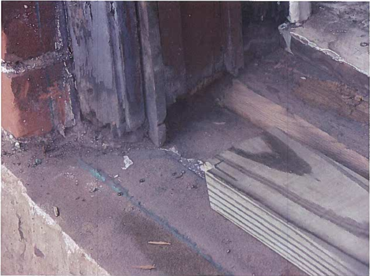
Figure 1: New pressure treated sill installed on Trolley Barn window 2004.
