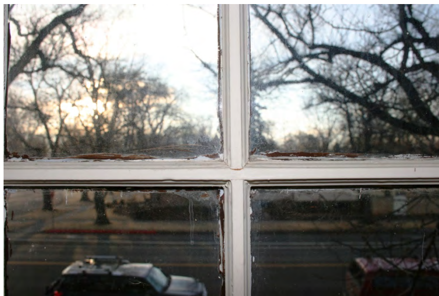
Image 2: Window 2-1, note the narrow muntin profile. This matches all of the other historic windows in the house
