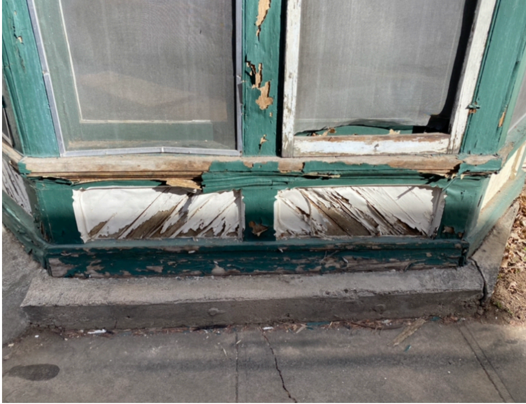
Base of south bay window
