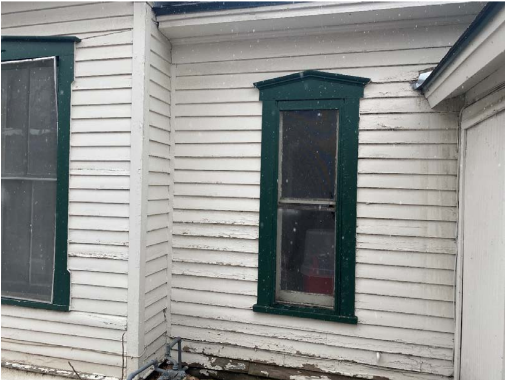
North elevation, hyphen, looking south.
