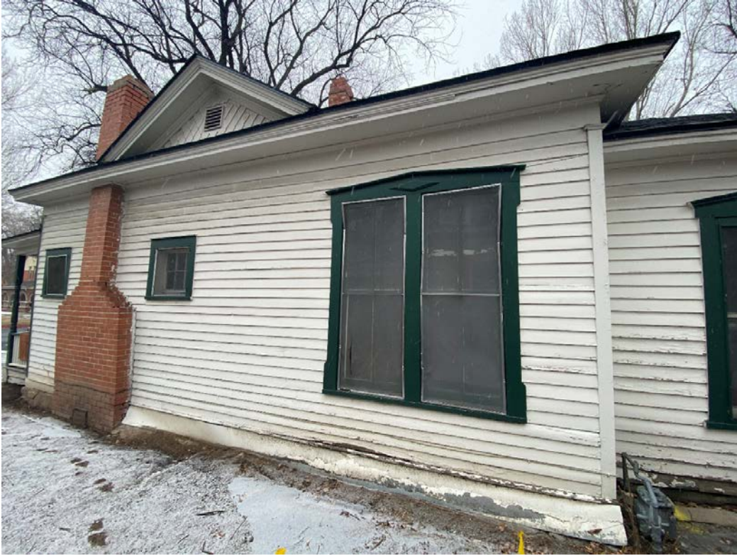
North elevation, front section, looking south.
