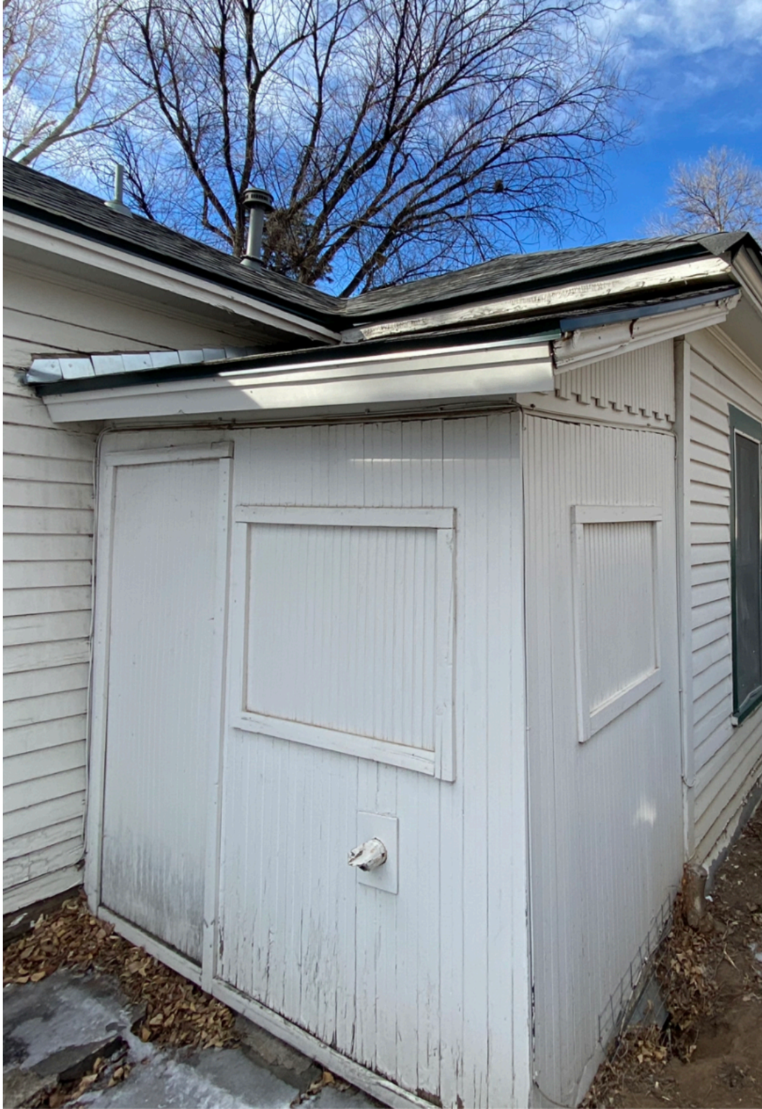
North elevation, rear section, looking southeast
