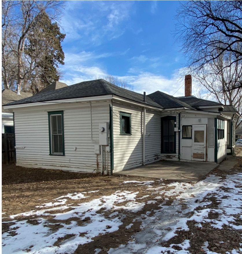
Rear elevation, showing location of addition, looking northeast.
