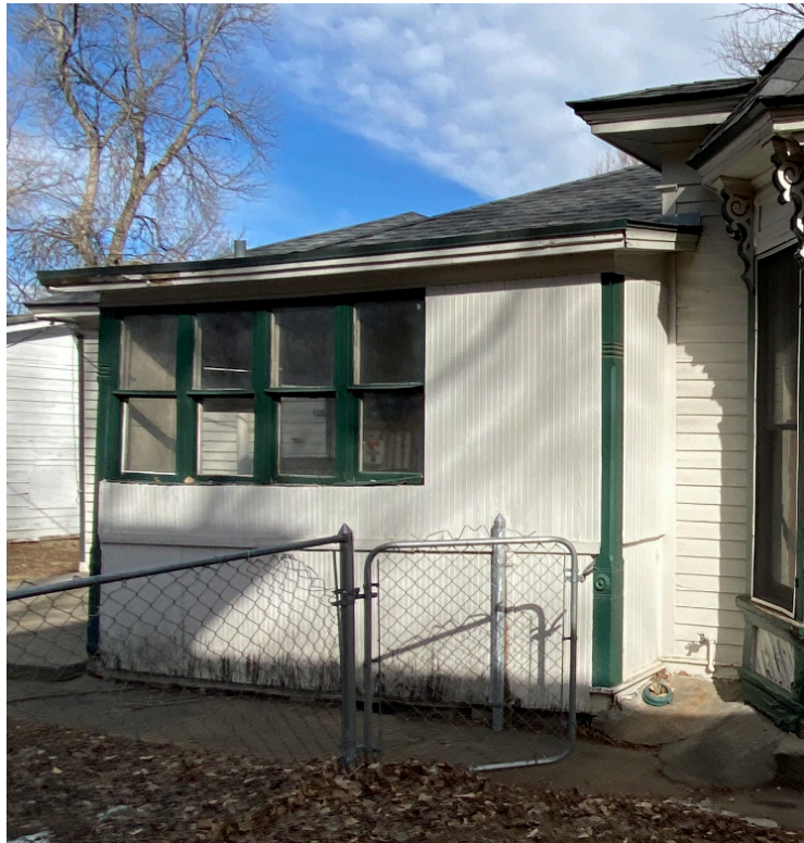
South elevation, rear portion, looking north
