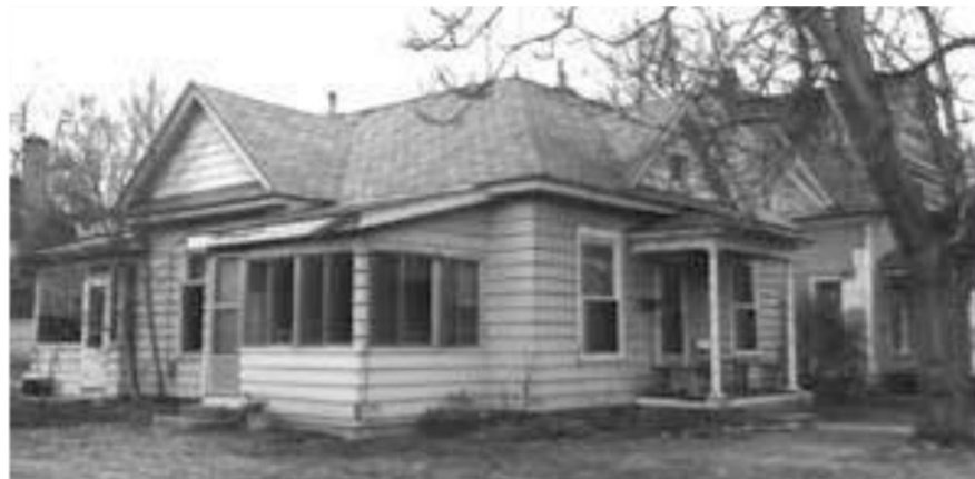
Kerrick Property, 1995, Historic Survey image, City of Fort Collins, https://fchc.contentdm.oclc.org/digital/collection/ph/id/12979 .
