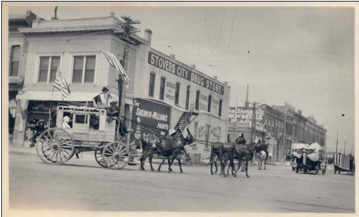
Figure 2: Circa 1914 photograph of 261 Linden Street showing painted brick facade.
