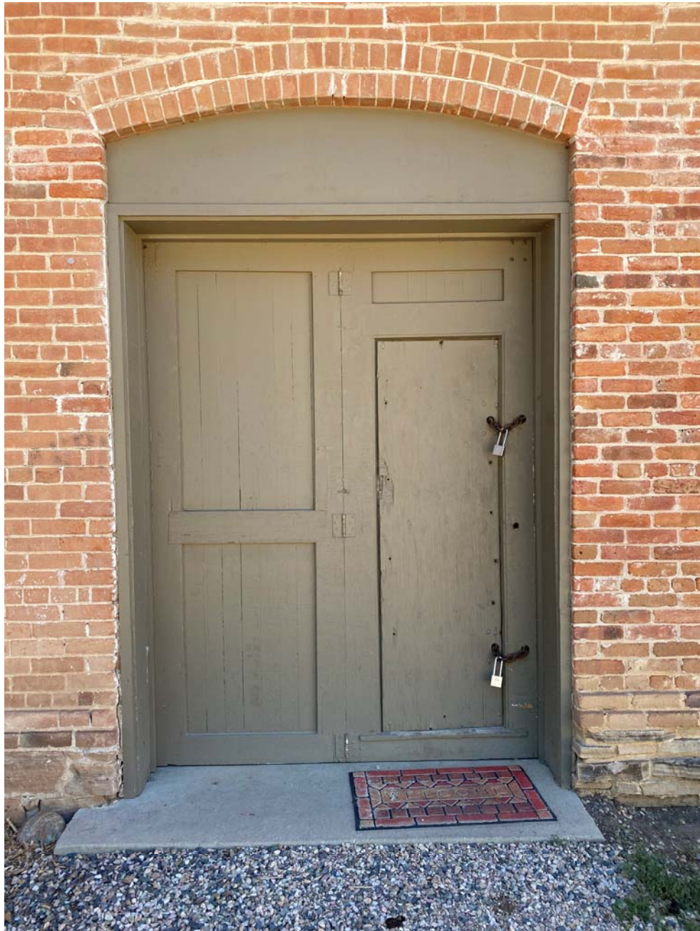
Picture 2- Elevation of Existing Door at the Filter Building
