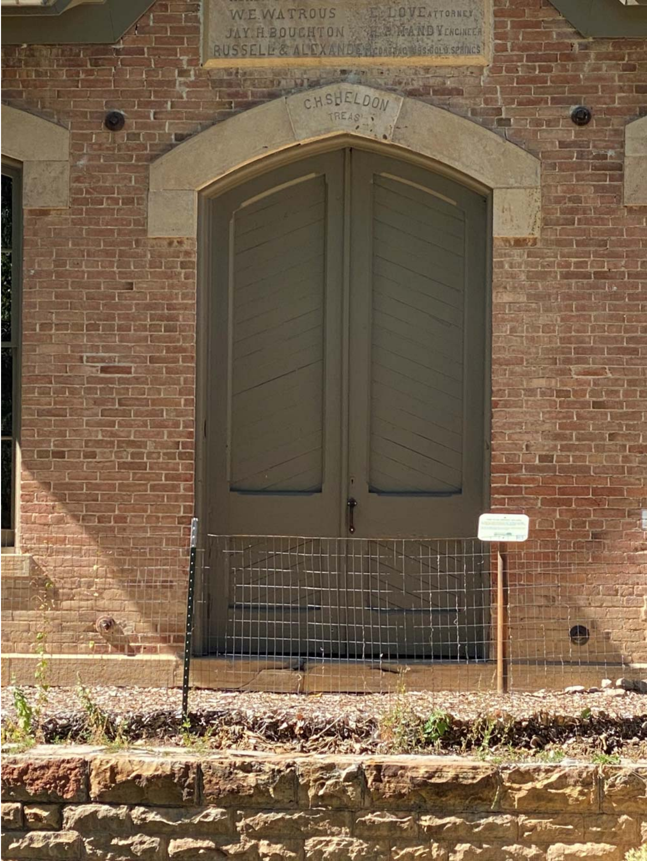
Picture 1-Elevation of Existing Door at the 1882-1883 Building
