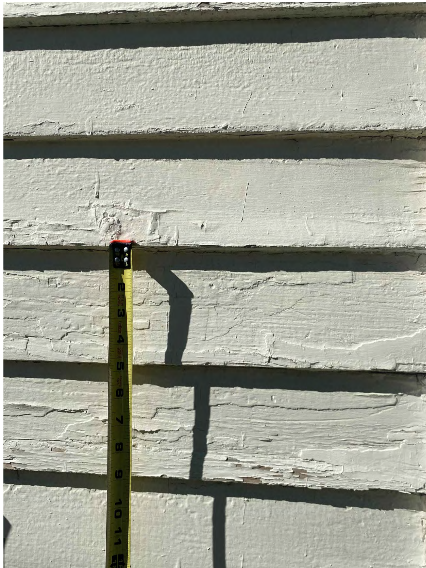
East Side lap siding, 5" exposure
