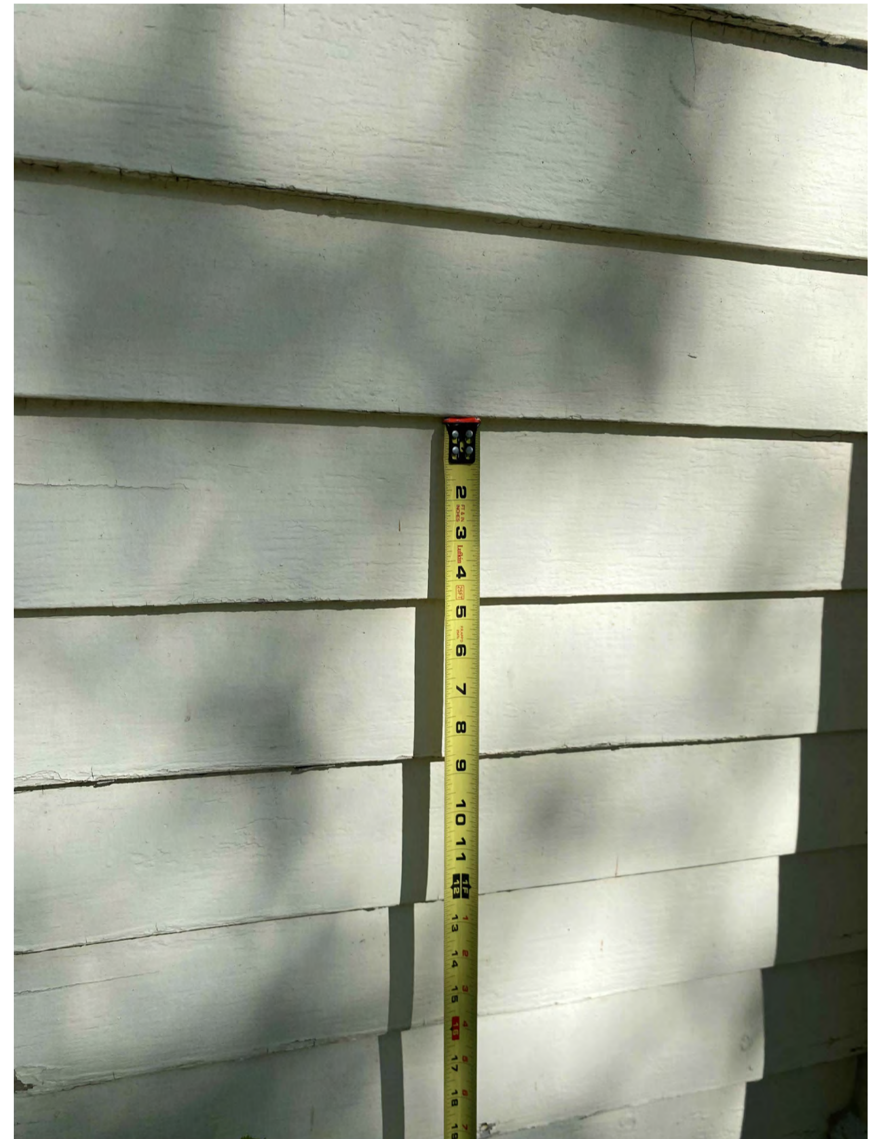
North Side lap siding, 5" exposure
