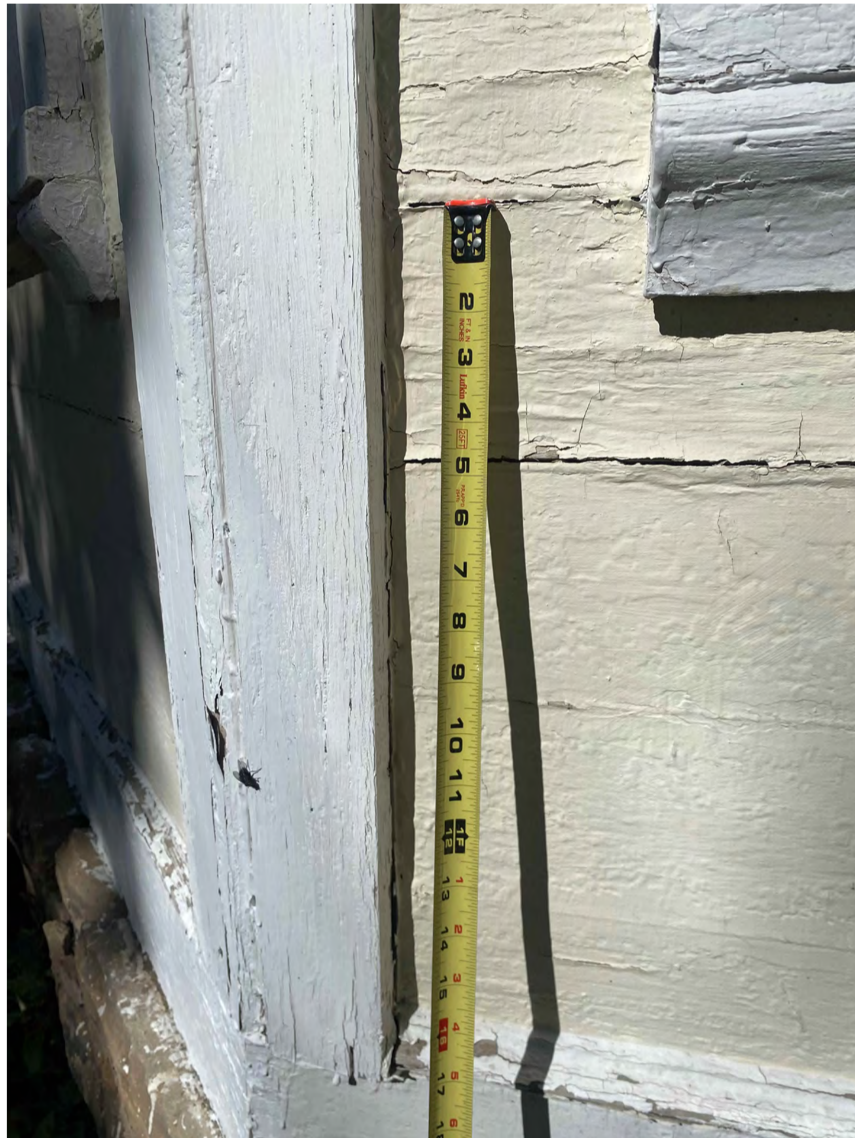
Front Bay Window in-plane siding, 5" exposure
