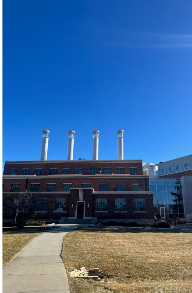
Fig 6: Sidewalk View of Powerhouse west
