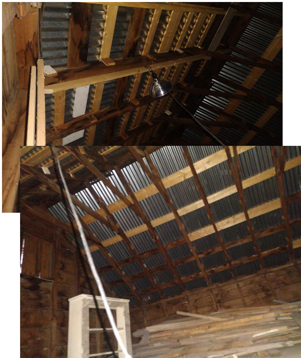
Figure 1: Existing Roof Framing
