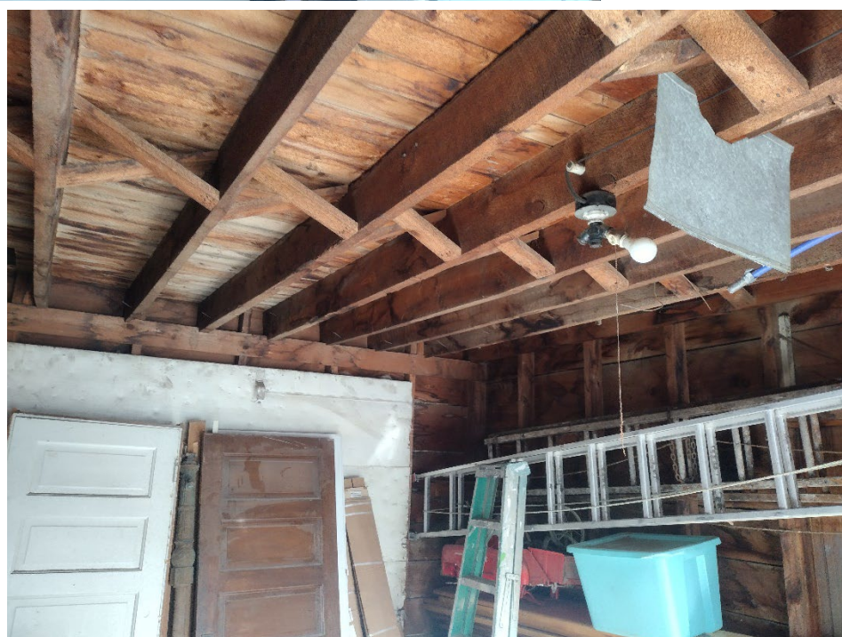
Figure 2: Existing Second Floor Structure
