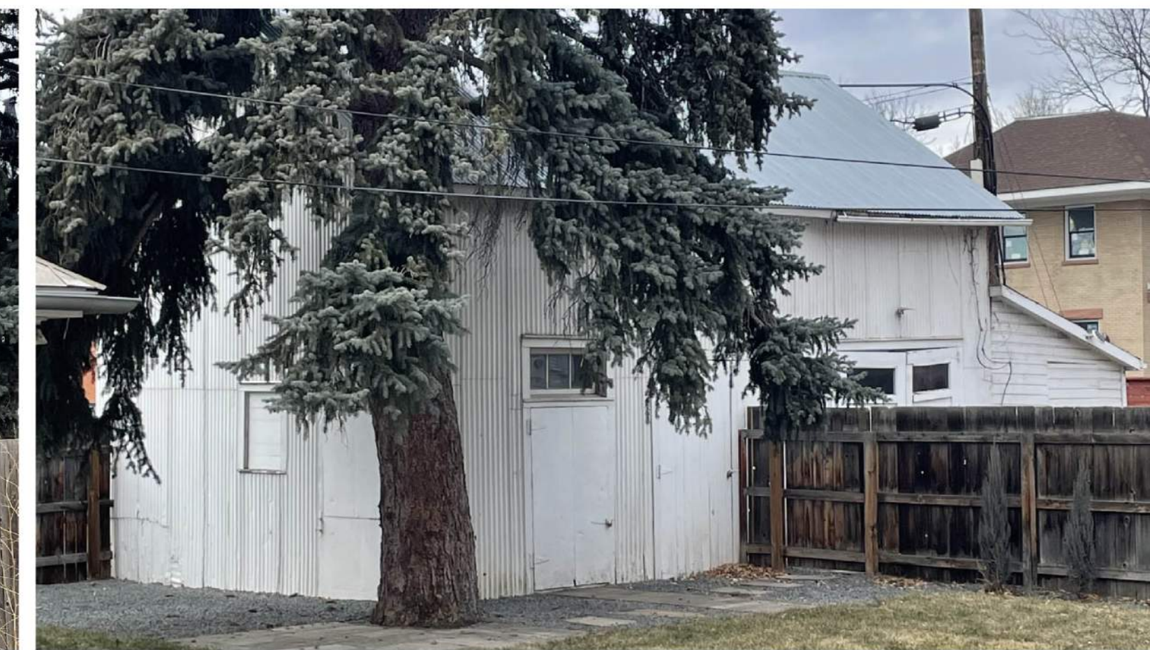
EXISTING BARN - SOUTHEAST CORNER
