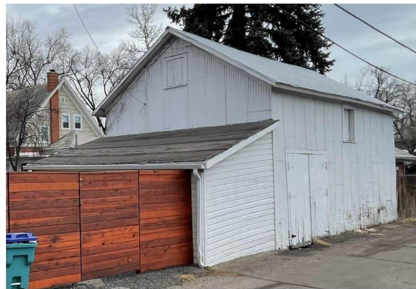
EXISTING BARN - NORTHWEST CORNER
