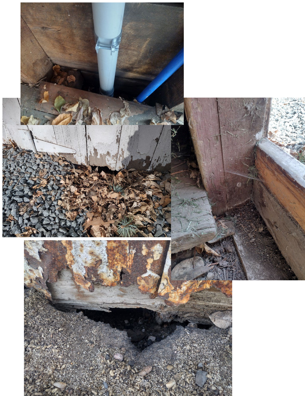
Figure 4: Base of Framing
