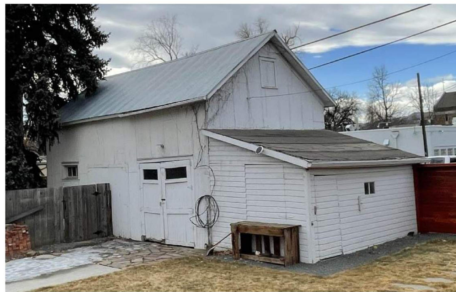
EXISTING BARN - NORTHEAST CORNER
