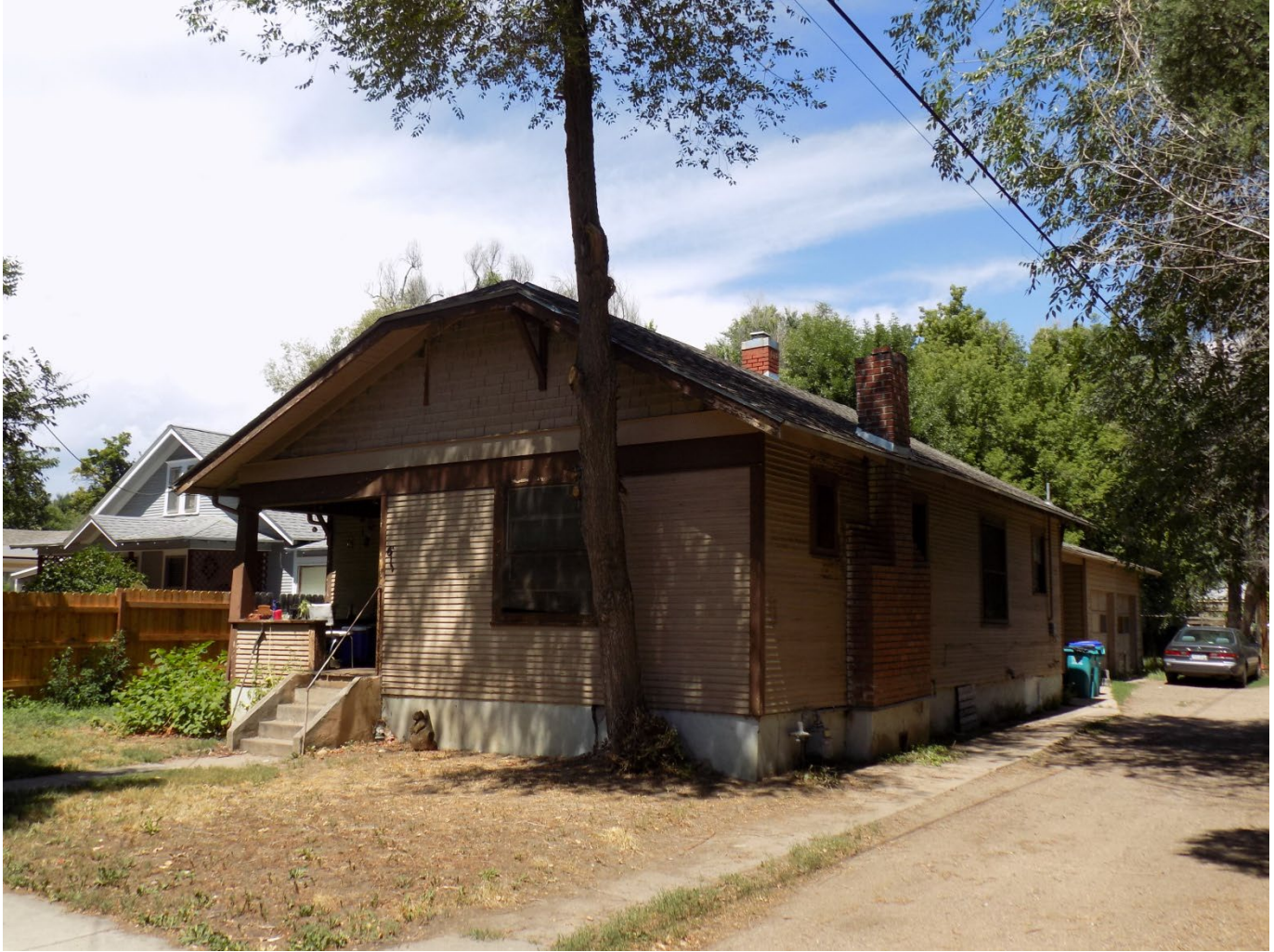
616 W Olive St., south façade and east side (Luke Anderson, August 2016)
