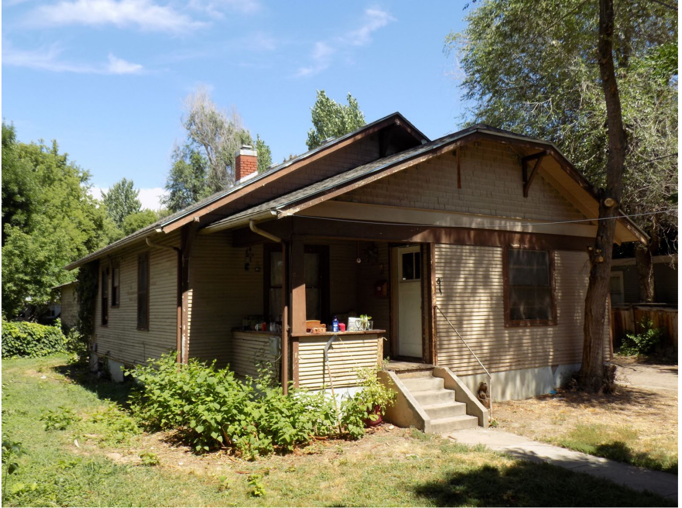
616 W Olive St., west side and south façade (Luke Anderson, August 2016)
