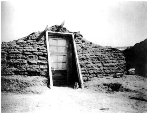
Figure 17. Sod schoolhouses, like this one in Logan County, Colorado, were common on the treeless plains of the state. ( Library of Congress )
