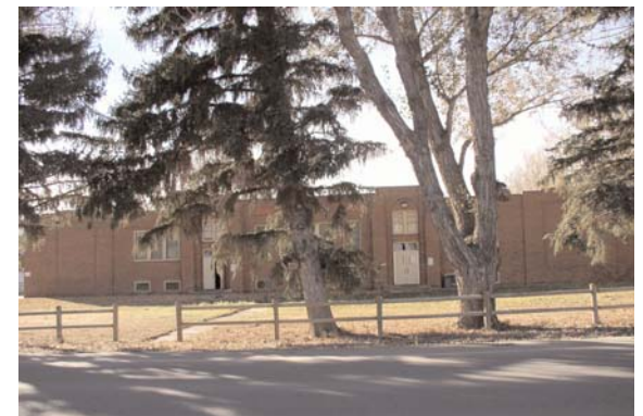
Figure 35. The Waverly School was a rather sophisticated and large building for its rural location. (Photo by the author)
