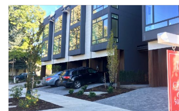
Tuck Under "$20,000 / space"
