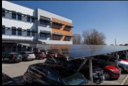
D. Parking lot solar panels
