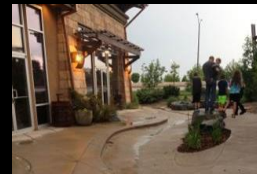
I. Paved drainage feature
