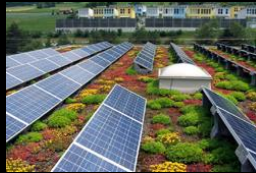
B. Solar green roof
