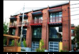
I. Lofts above workshop space
