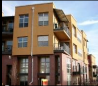
D. Stacked units
