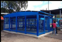
H. Secure/covered parking (self-serve)
