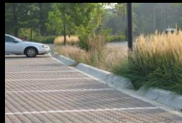
H. Porous pavers in parking areas
