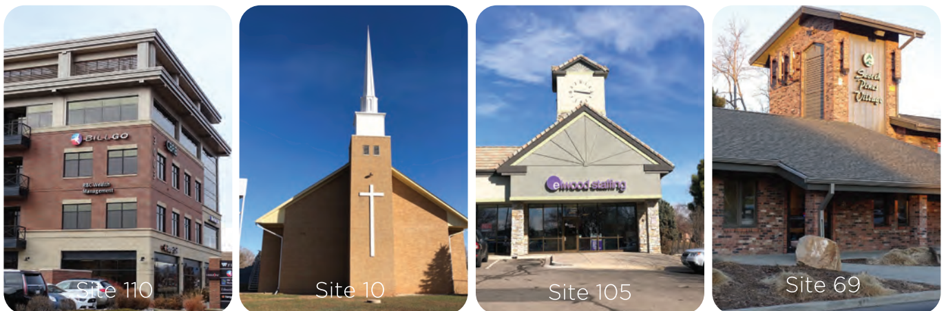
Figure 5: Concealed and Semi-Concealed Base Stations
