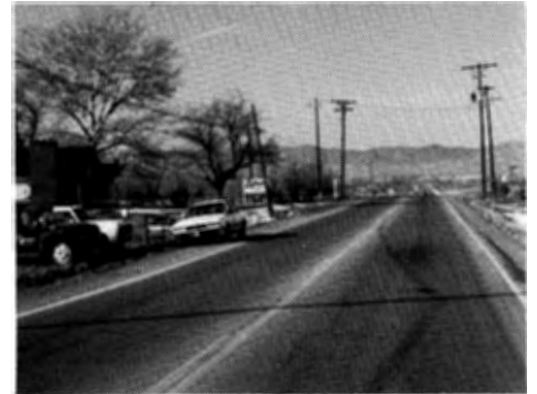
Overhead Power Lines
