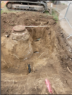
Crews removed an old brick sewer manhole
